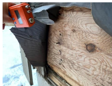
Photo 30: Close-up view of opening.
