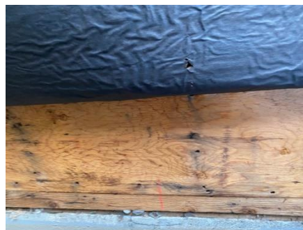
Photo 16: Close-up view of opening.
