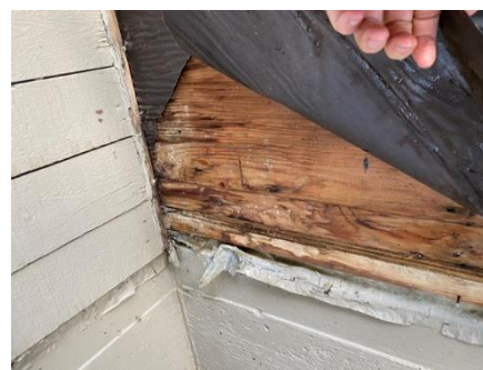
Photo 26: Close-up view of opening.
