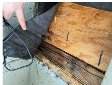
Photo 18: Close-up view of opening.
