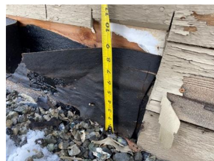
Photo 6: Close-up view of opening.
