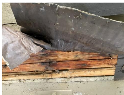
Photo 14: Close-up view of opening.
