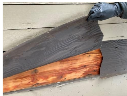
Photo 12: Close-up view of opening.
