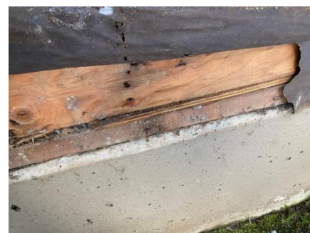
Photo 10: Close-up view of opening.
