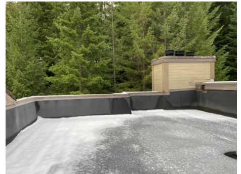
Photo 2: Fifth floor roof.
