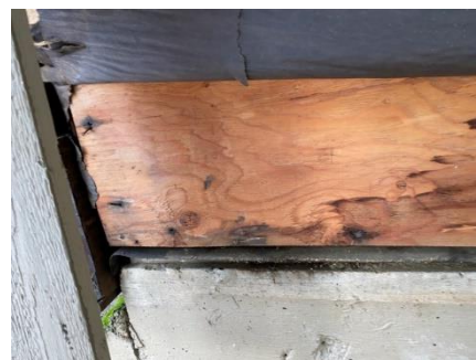
Photo 4: Close-up view of opening.
