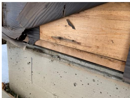
Photo 2: Close-up view of opening.
