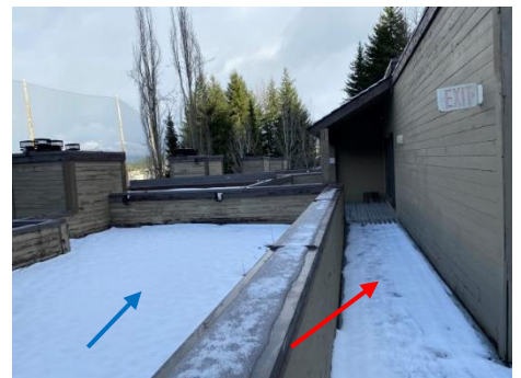
Photo 3: Roof deck (red arrow) and adjacent flat fourth floor flat roof (blue arrow).
