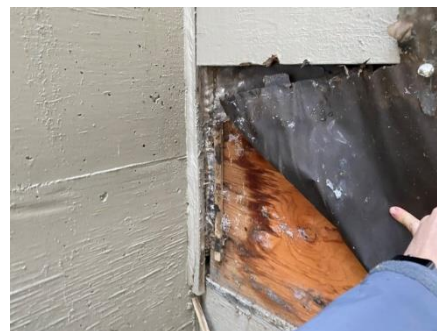
Photo 32: Close-up view of opening.
