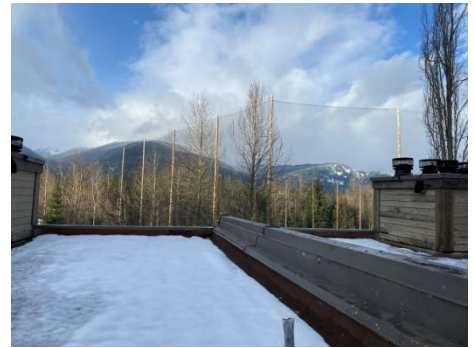
Photo 4: Fourth floor roof.
