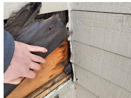
Photo 8: Close-up view of opening.
