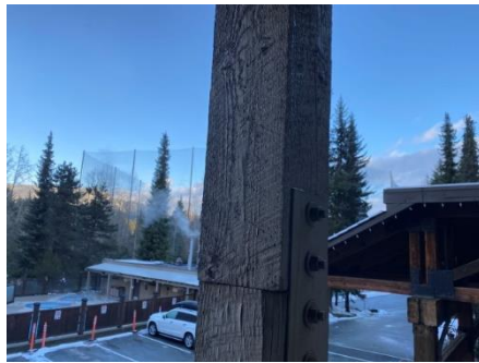
Photo 37: Balcony post splice mid-height.
