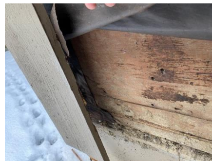
Photo 28: Close-up view of opening.
