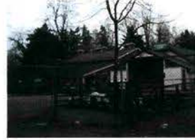
10. VIEW TOWARDS MAPLEWOODS FARM AND PARKING LOT
