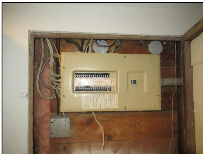
12. Main electrical disconnect
