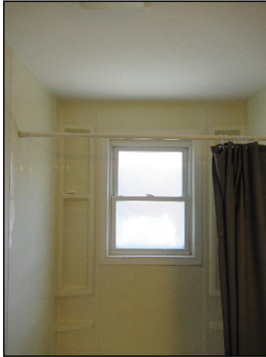
48. Lost seal on double glazing
