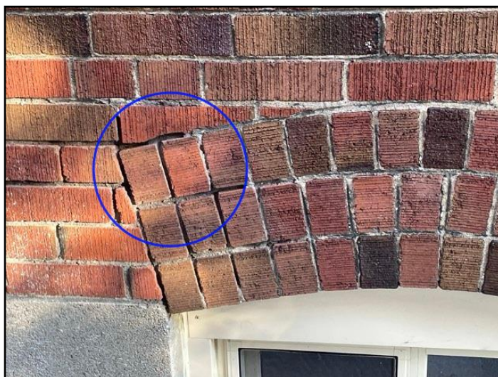
Mortar deterioration
