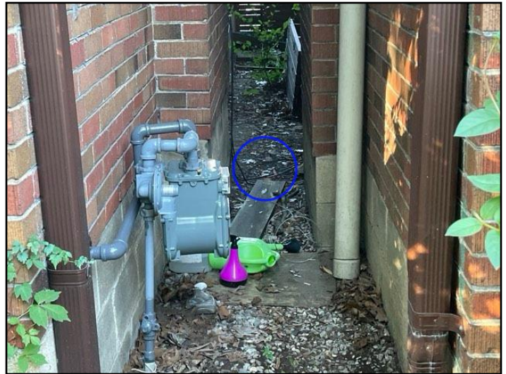
Elevated moisture Left side basement bedroom
