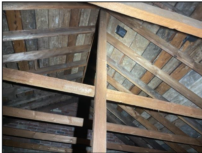
Rafters/ceiling joists
