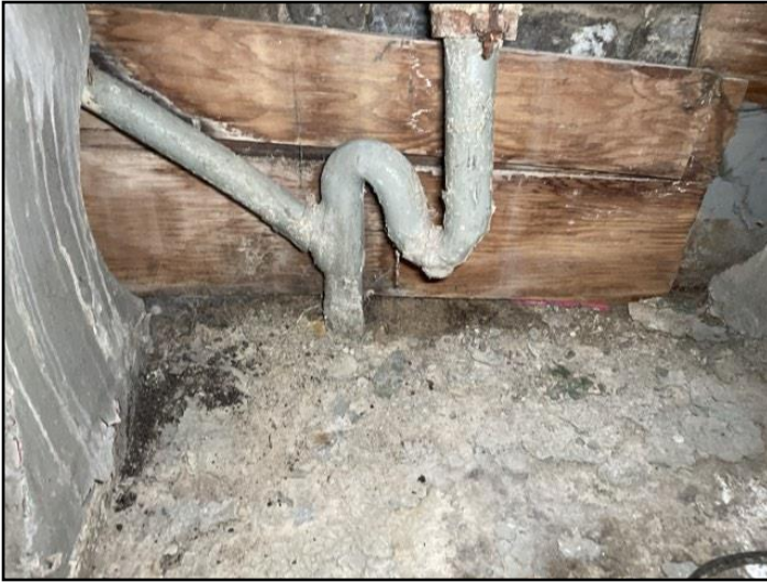
Hand formed lead drain
