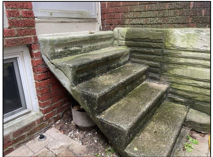
Gutter is leaking in this area
