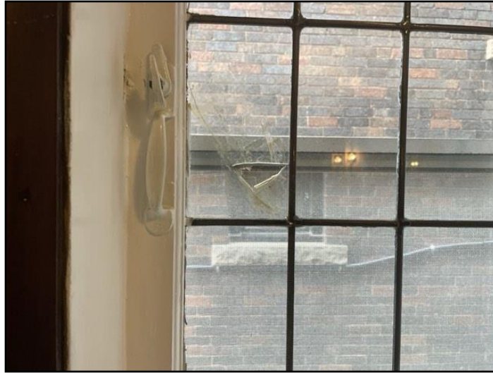
Cracked-Stairwell window
