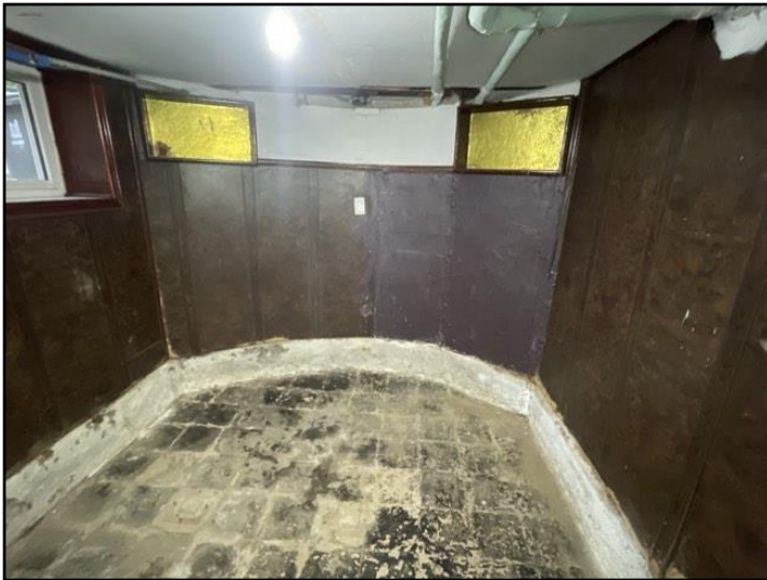
Rear addition basement
