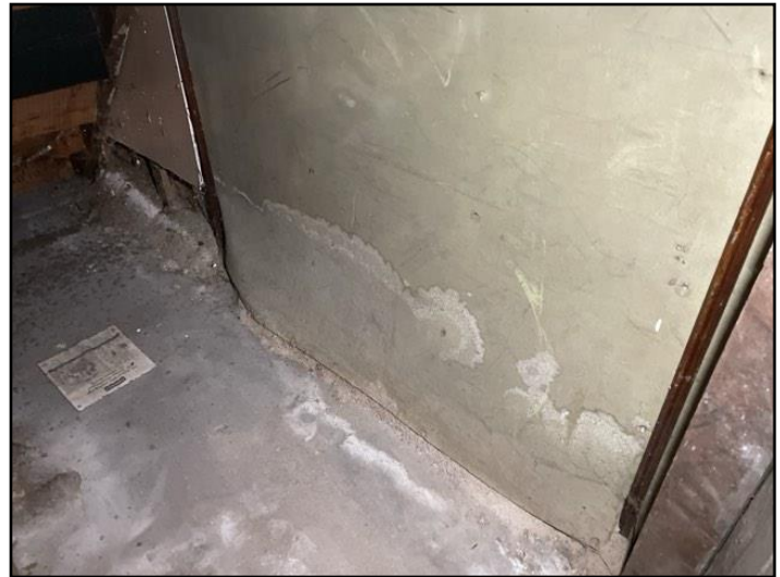
Below basement stairs - Left side
