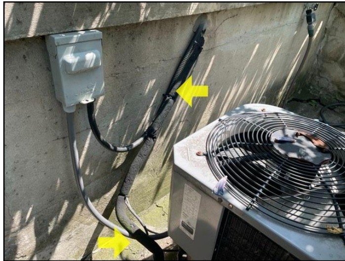
Insulation - deteriorating
