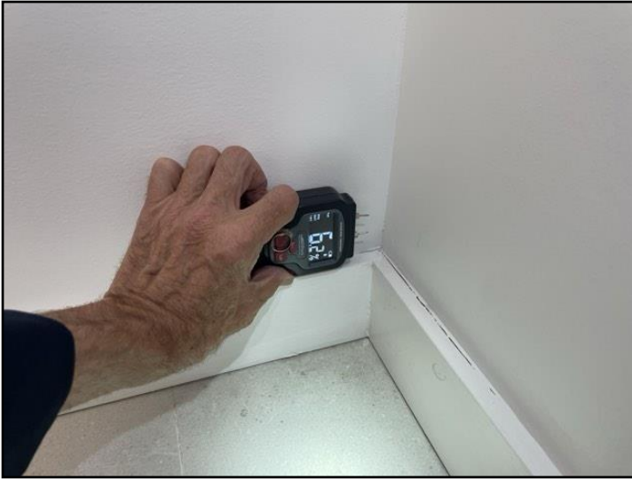
Right Wall, Rear Room
