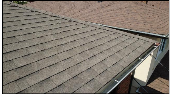
Asphalt shingles
