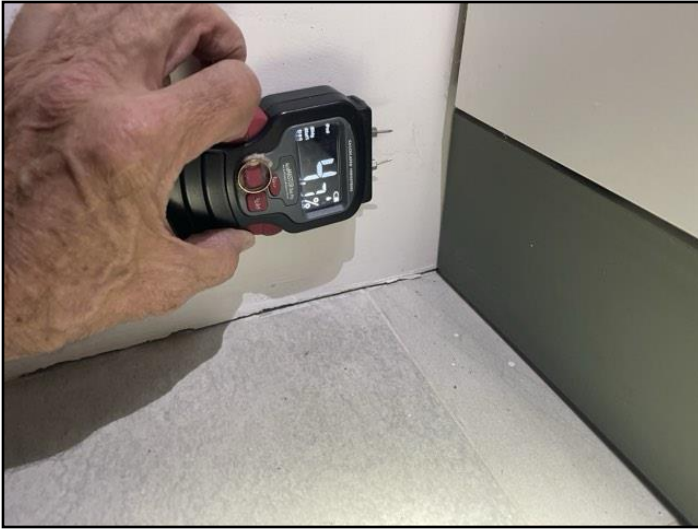
Right Side (Furnace Room)
