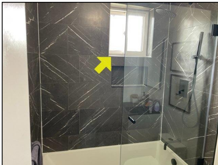
Window in shower enclosure
