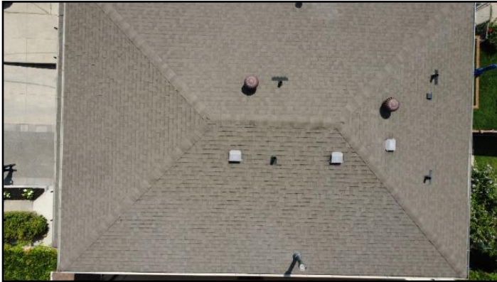
Asphalt shingles
