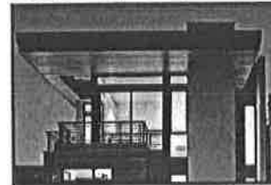
Street Side Deck
