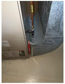
()Recommend cleaning or changing on a monthly basis to ensure life of furnace or follow recommended manufacture instructions of unit or filter .Installing of the filter in the correct direction is important.
