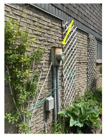
()Digital meter 200amp service from city 240 volt 1 phase, 3 phase. Top of unit rusted.
