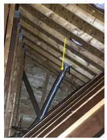
Exhaust venting for the bathroom has insulation missing. It is recommended to install insulation on the pipe to Consult a qualified contractor.
