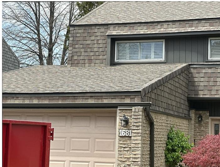
( )Shingles are in good condition in visible areas only at time of inspection unless noted. Continue a yearly checkup and regular maintenance to prolong the life of the roof.
