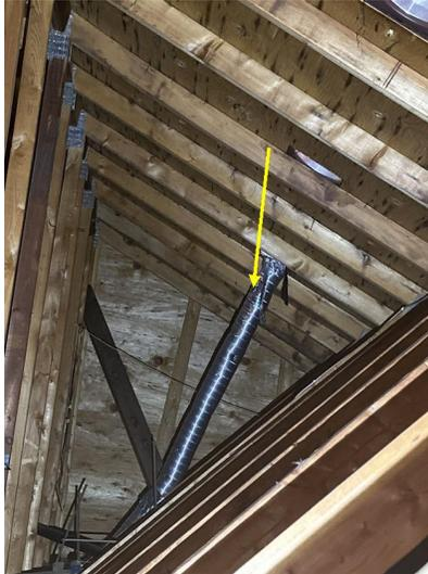
Exhaust venting for the bathroom has insulation missing. It is recommended to install insulation on the pipe to Consult a qualified contractor.
