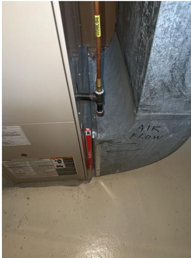
()Recommend cleaning or changing on a monthly basis to ensure life of furnace or follow recommended manufacture instructions of unit or filter .Installing of the filter in the correct direction is important.
