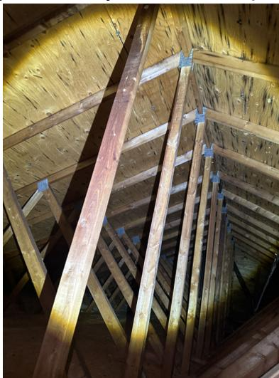
Nail staining noted. Dry at time of inspection.
