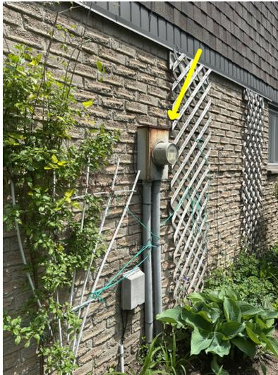
()Digital meter 200amp service from city 240 volt 1 phase, 3 phase. Top of unit rusted.
