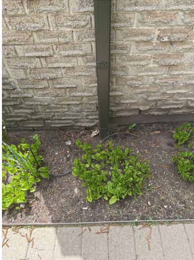
(())It is recommended to provide downspout extension 4 to 6 feet away from the home for proper water drainage.
