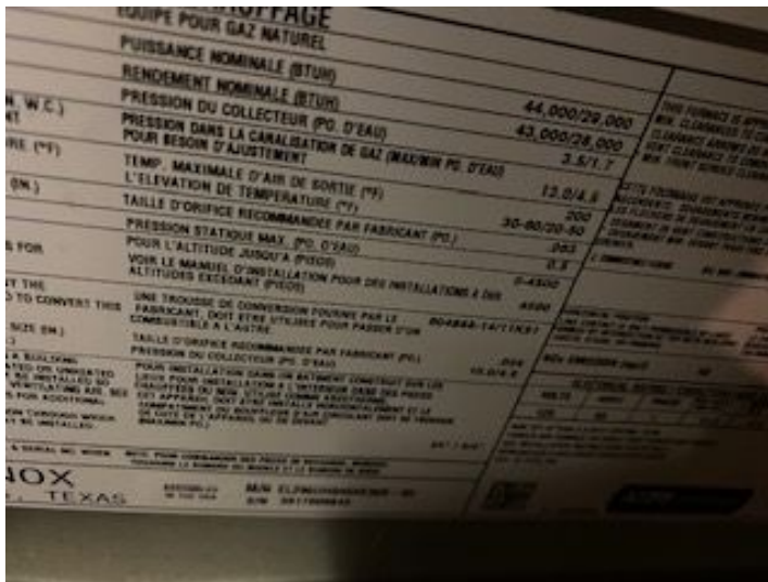
( ) Annual preventive maintenance is recommended.
