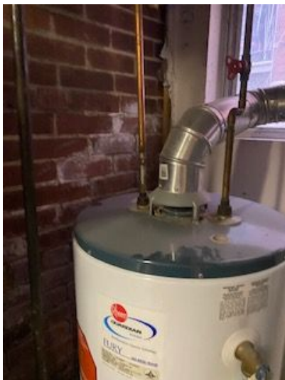
( ) No bonding wire (not visible noted at time of inspection) from gas line. Correction is needed. Consult a qualified contractor.
