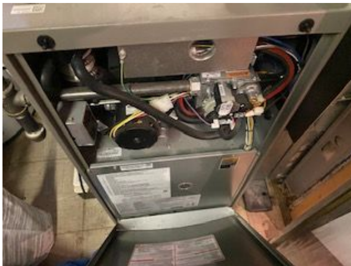
( ) Annual preventive maintenance is recommended.
