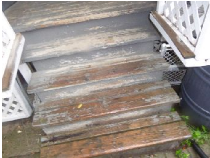
( )Safety railing is recommended.
