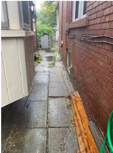
heaved/settled areas observed.
