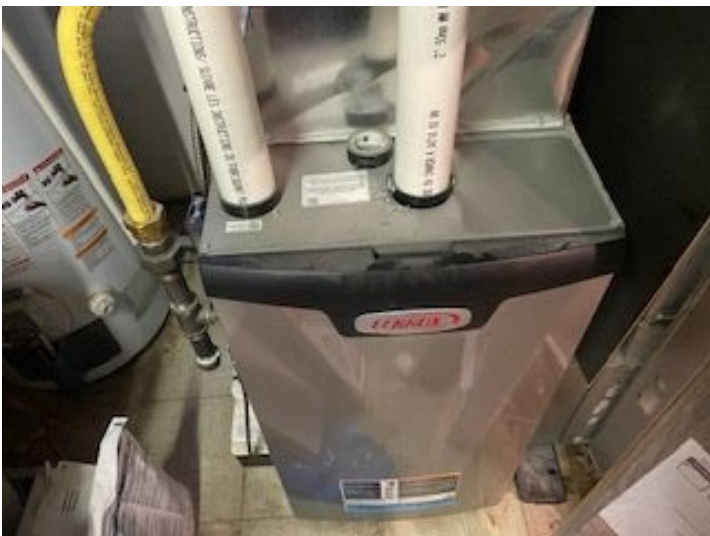
( ) Annual preventive maintenance is recommended.
