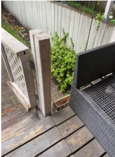
no fence noted
