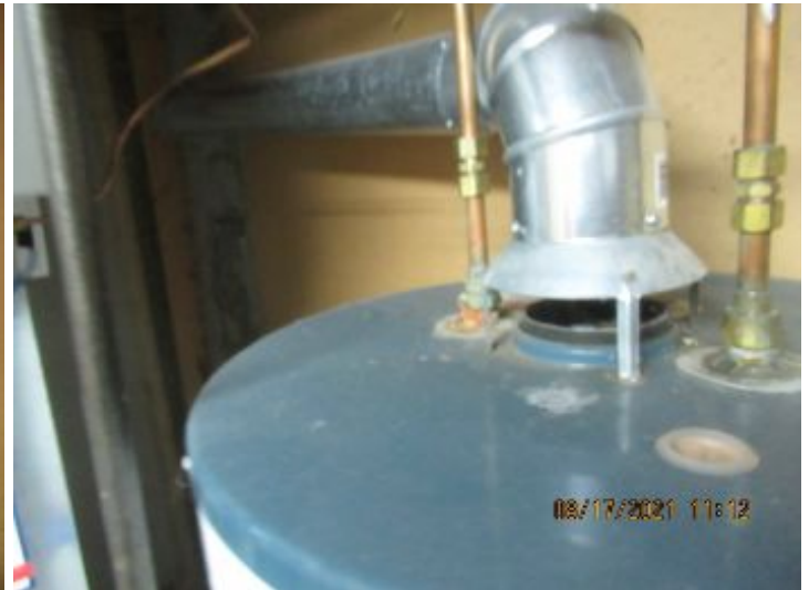
()It is recommended not to store items near the hot water and furnace area for safety and access entry.
