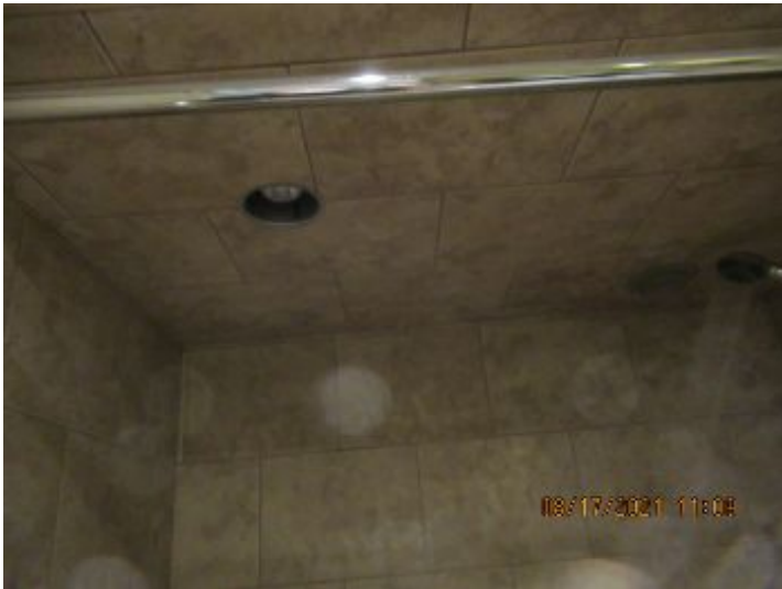
washroom lights in bathroom not coming on
