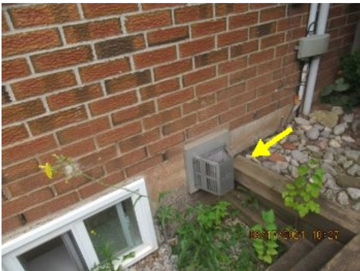
exhaust is close to the wood, not within standard
