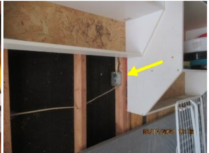
Cover plate needed for safety.
