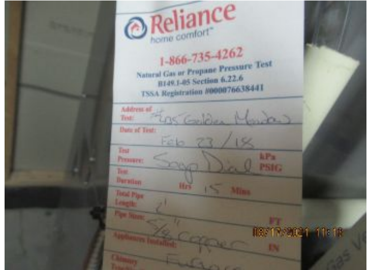
( ) Annual preventive maintenance is recommended.
