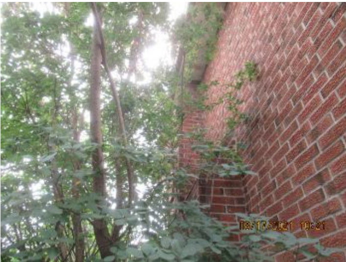
( )Suggest trimming back vegetation from brick,vinyl etc cladding- home to prevent deterioration.
