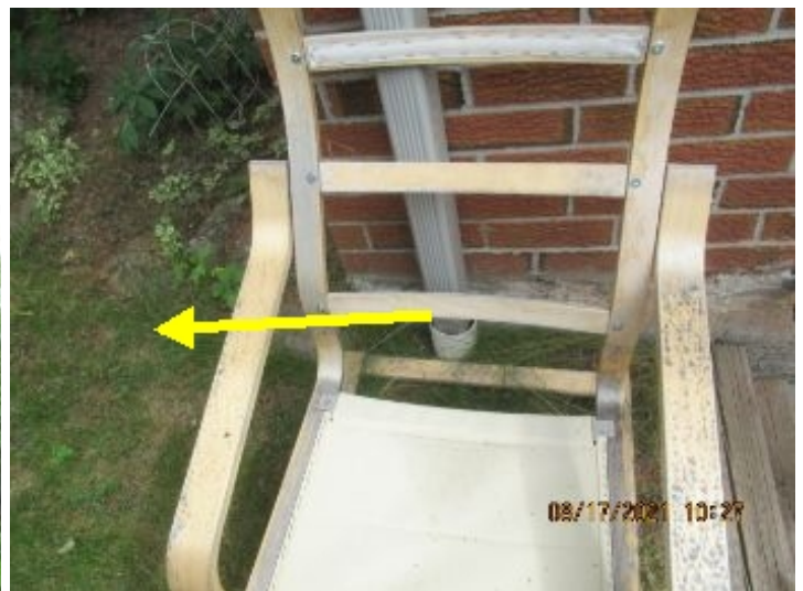
( )It is recommended to provide downspout extension 4 to 6 feet away from the home for proper water drainage.
