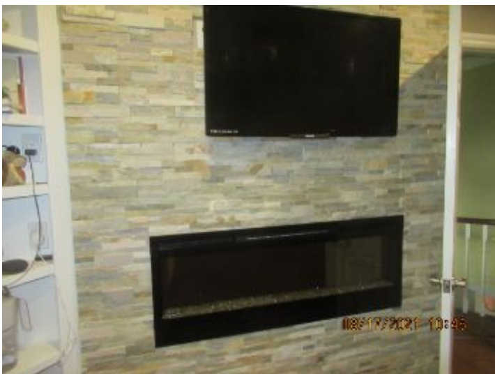
( )Yearly inspection- cleaning is recommended for maintenance. Consult a qualified contractor. Safety is needed for young children.
