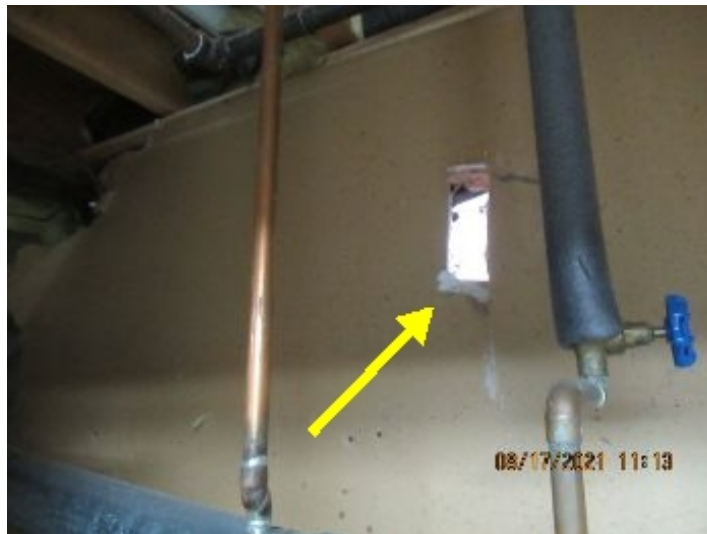
blocked window in the furnace room
