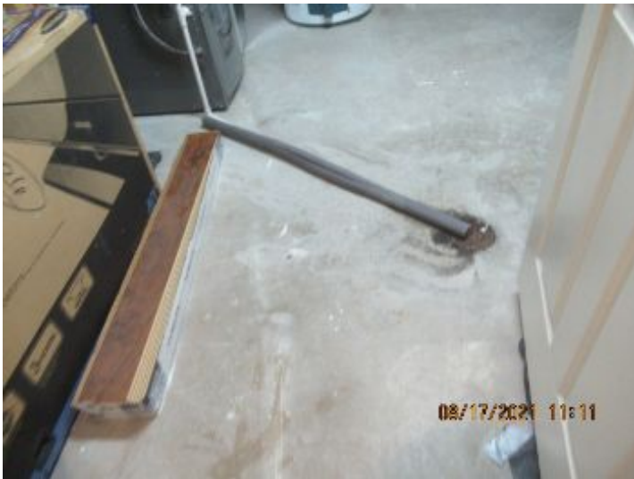
( )Basement floor drain. It is recommended never to cover the floor drain for safety and emergency purposes.
