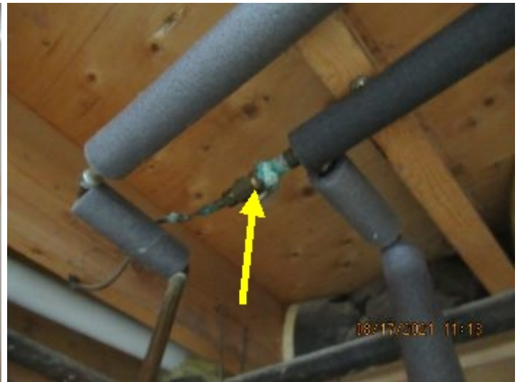
aged, furnace room
