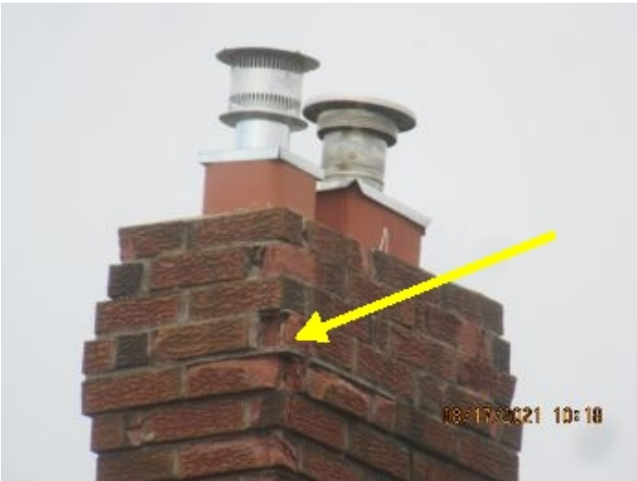
( )Brick and mortar deterioration observed; repair advised. Consult a qualified contractor.
