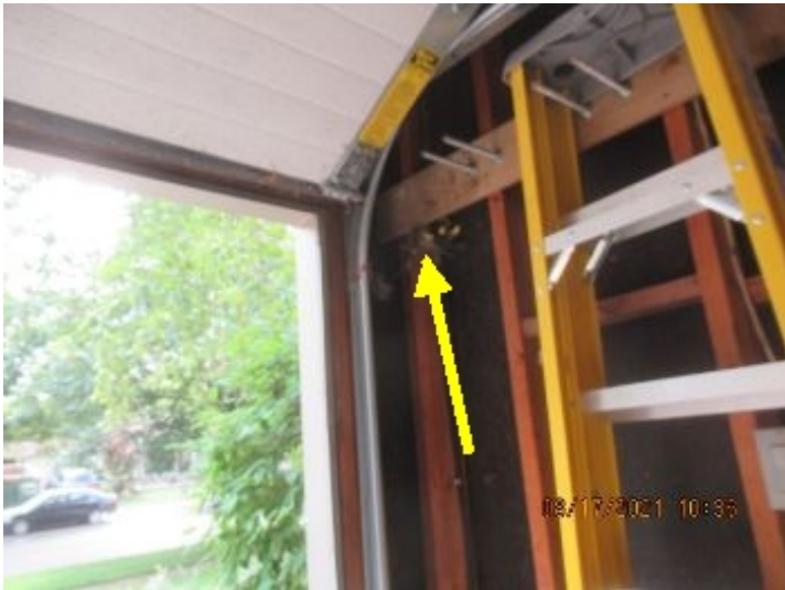
Cover plate needed for safety.
