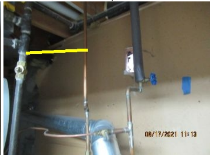
()No bonding wire (not visible noted at time of inspection) from gas line. Correction is needed. Consult a qualified contractor.
