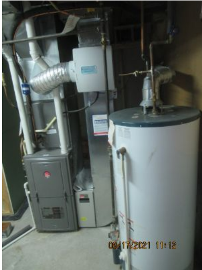
( ) Annual preventive maintenance is recommended.
