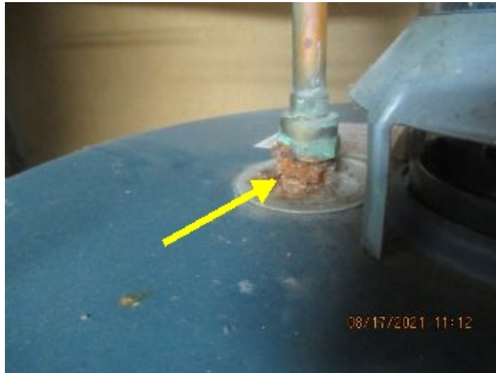
Corrosion noted at fittings, consult a qualified contractor.
