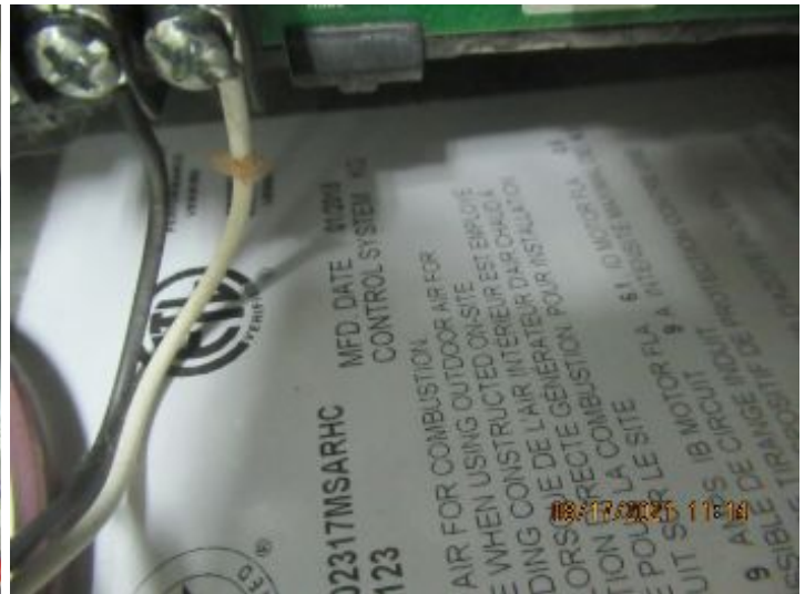
( ) Annual preventive maintenance is recommended.
