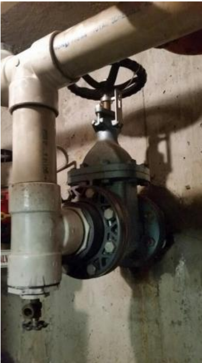
Domestic water pipes are WHITE. The shutoff valve is a black 'steering wheel' mounted horizontally above the white pipes, at the back of the sprinkler room, against the far wall.
