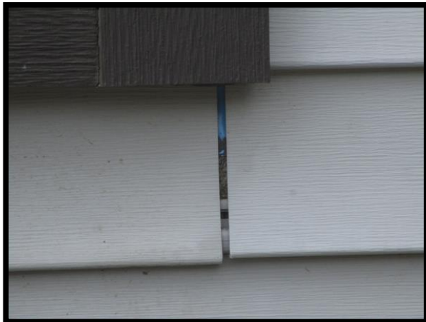
Seal siding joints
