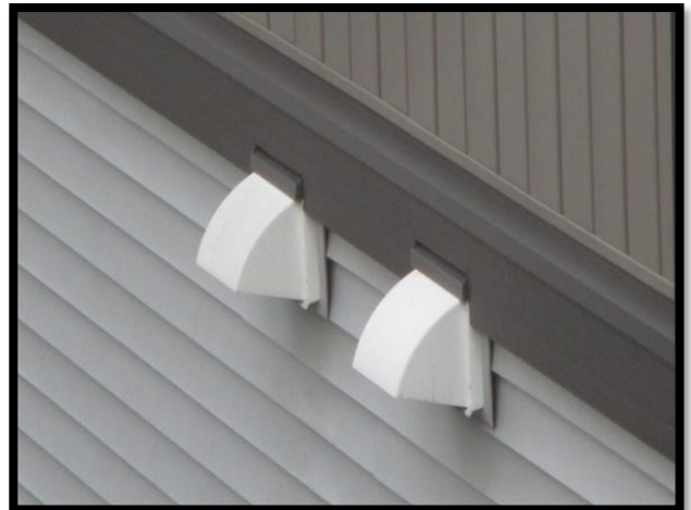
Vent covers/flashings
