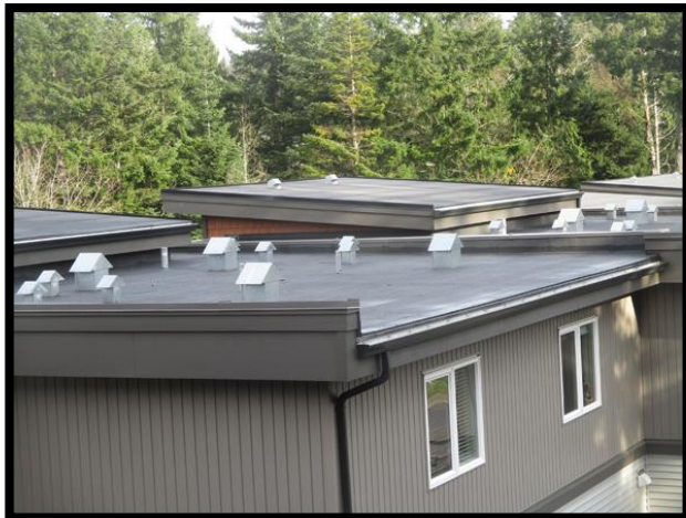
Roof membrane / vents
