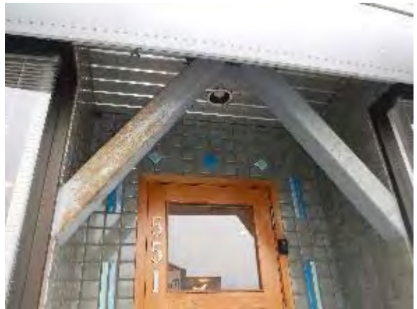
12–Exterior Coatings- metal structural supports
