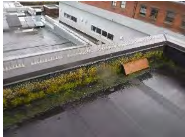
25-Areas of moss growth on SBS membrane at roof. Loose objects on roof.
