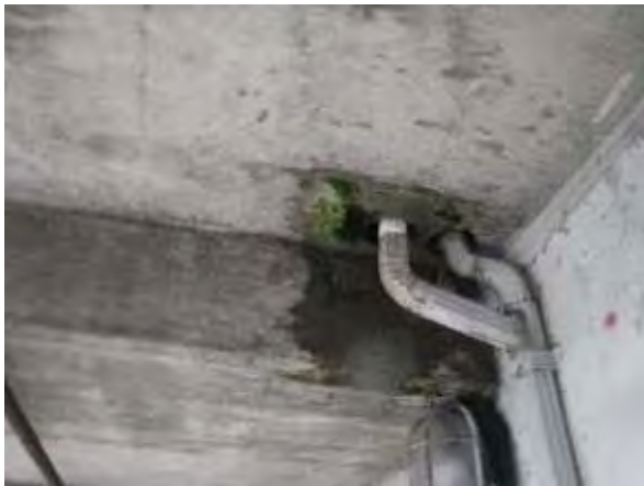
5 – Water leaking over light fixture
