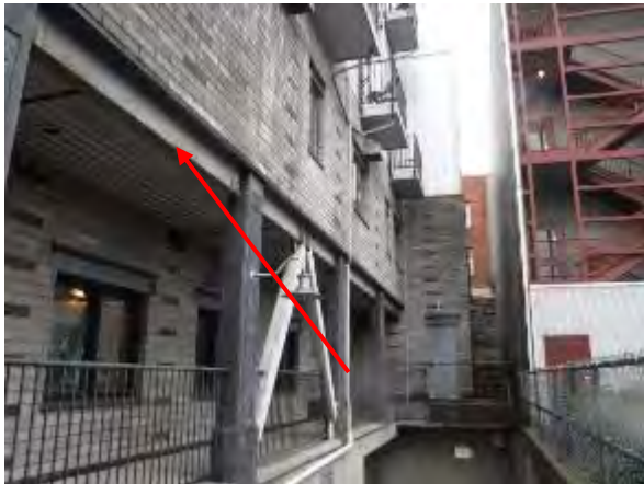
12-Exterior Coatings- metal structural supports
