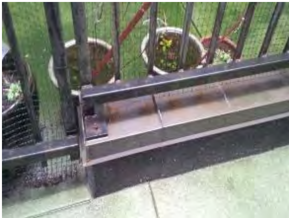
8– Railing repainting- rust noted on rails.
