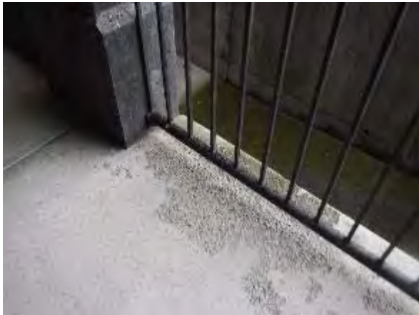
53 – Concrete scaling at pavement surface.
