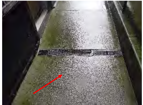
53 – California grate requiring repair
