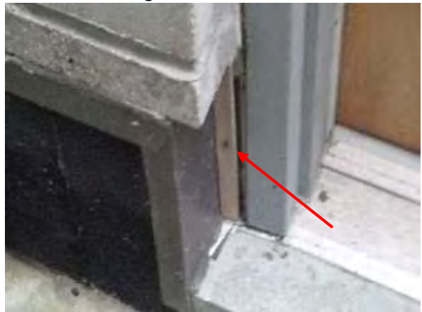
6 – Brick Cladding – Cladding missing at base of wall.
