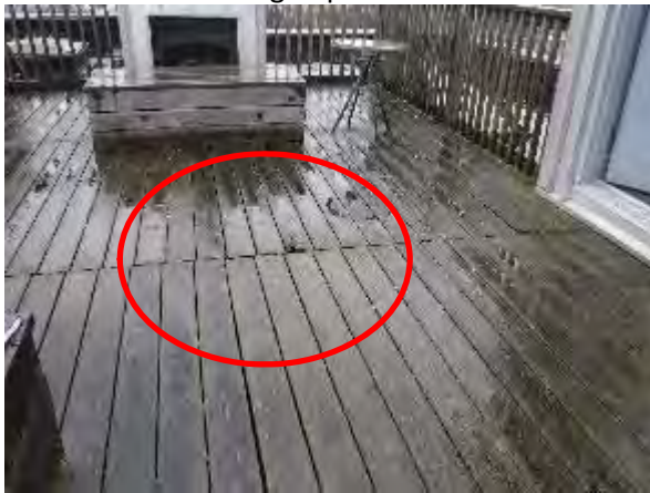
57 – Exterior wood decks -repair
