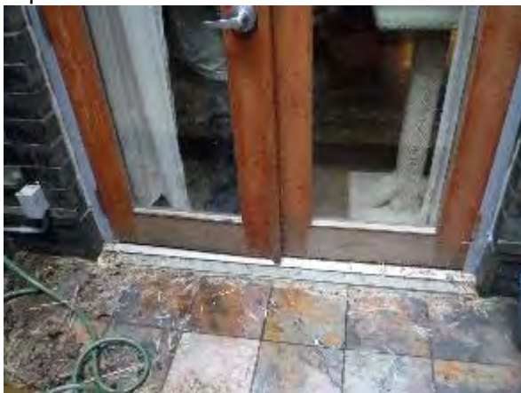
18- Wood finishes on double swing doors
