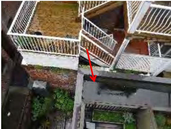
25 – Second floor roof deck area pooling water.
