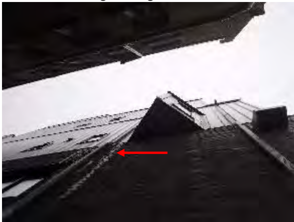
6 – Brick Cladding – Water saturation from water leaders
