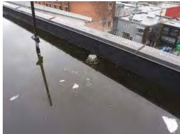
25- Pooling on roof due to blocked drain.
