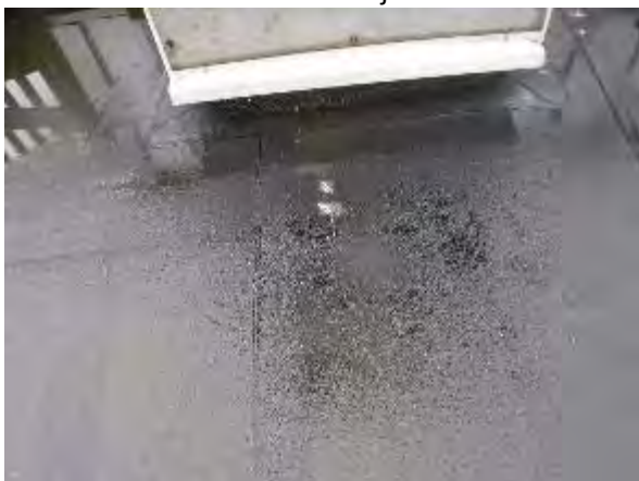
25-Degranelation of roof membrane
