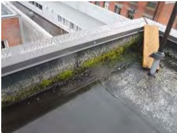
25-Areas of moss and lichen growth on SBS membrane at roof. Loose objects on roof.
