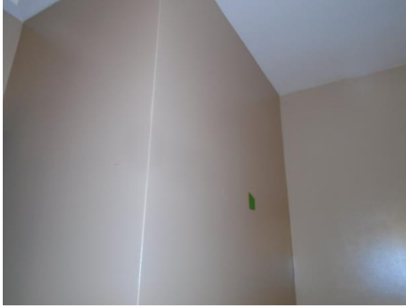
Photo 1: Smooth Plaster [2 layers] – Bathroom Wall (none detected)
