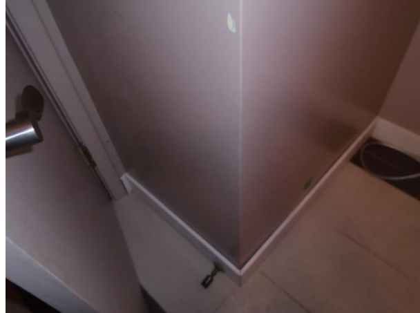
Photo 2: Smooth Plaster [2 layers] – Bathroom Wall (ND)
