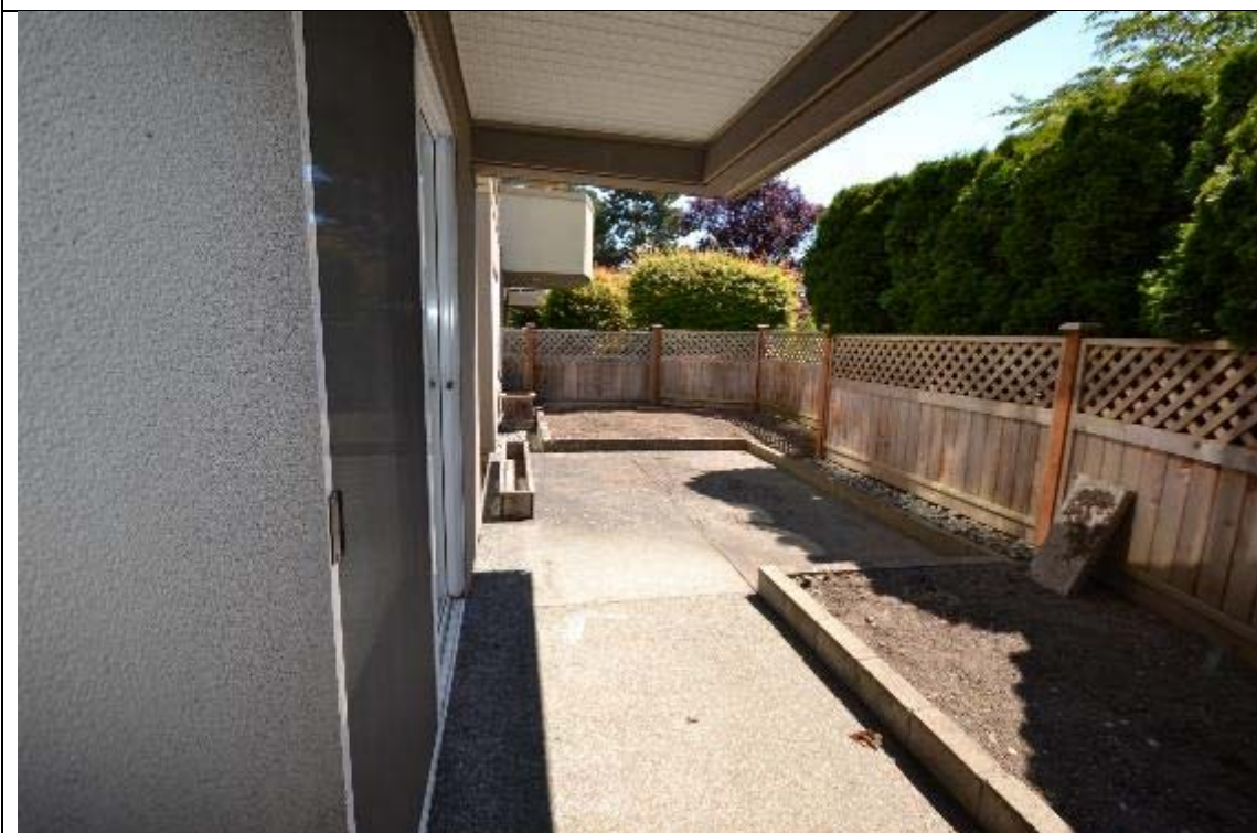
View of Patio Fencing
