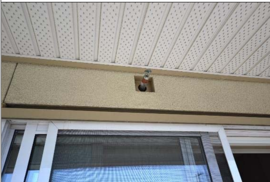
Exterior Sprinkler Head
