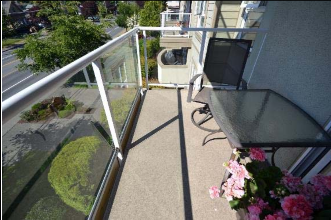
View of Typical Balcony Membrane
