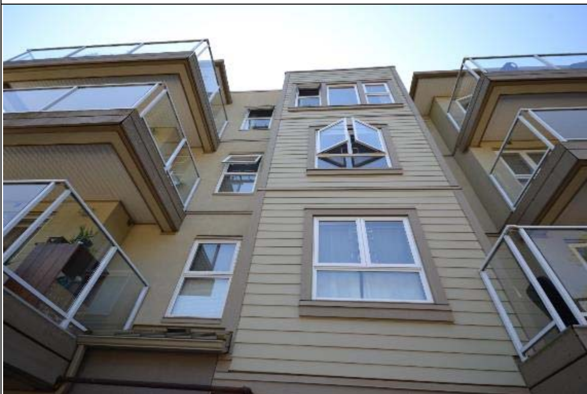
View of Fibre Cement Siding
