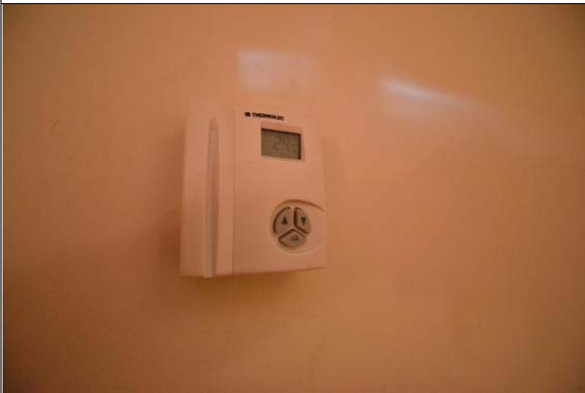
New Thermostat for RTU
