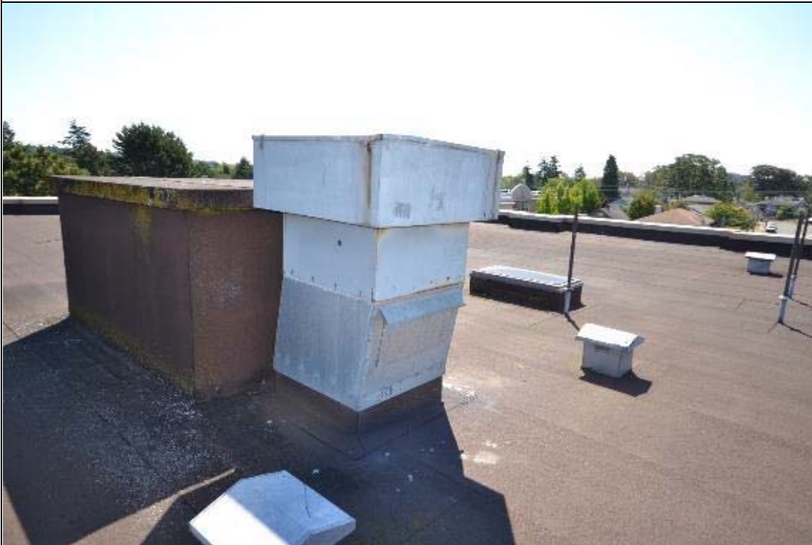
Rooftop Make Up Air Unit
