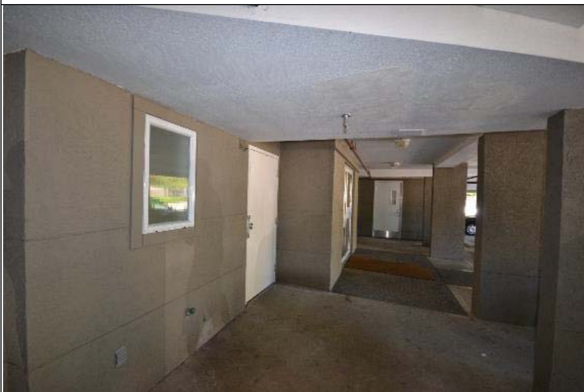
View of Original Stucco
