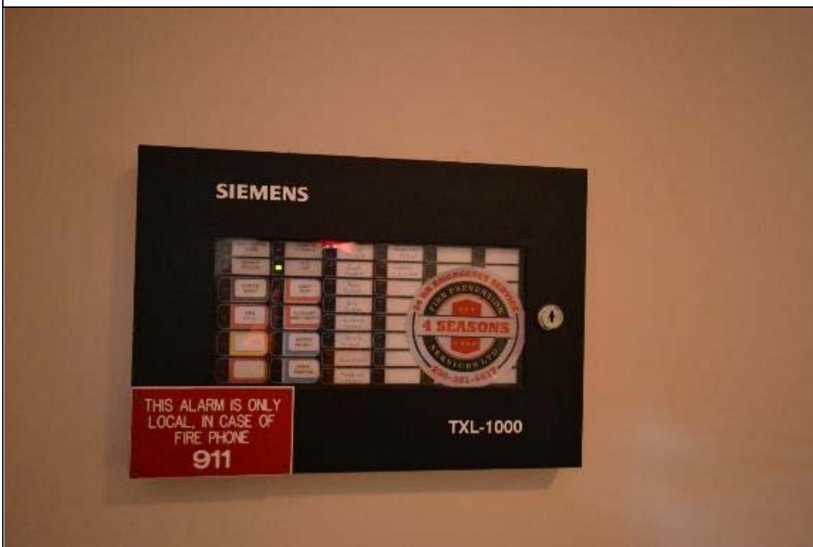
Fire Alarm Control Panel
