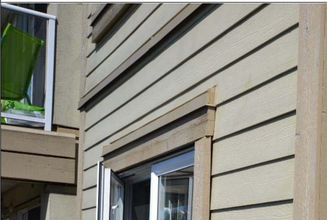
Paint Showing Deterioration and Wood Beginning to Cup/Crack
