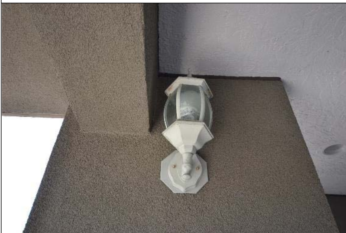
Exterior Light Fixture
