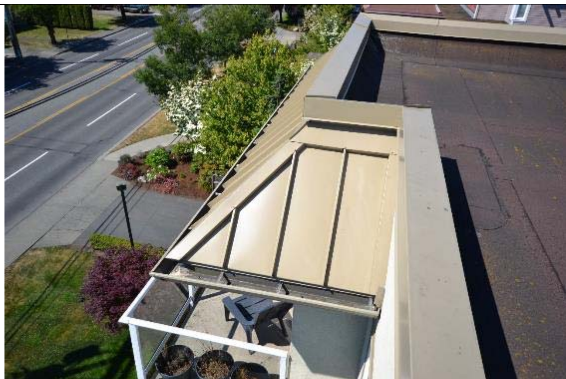
View of Roof
