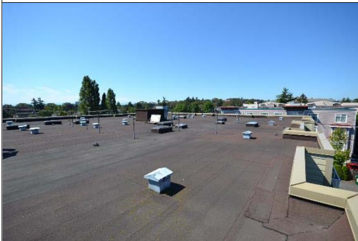
View of Roof
