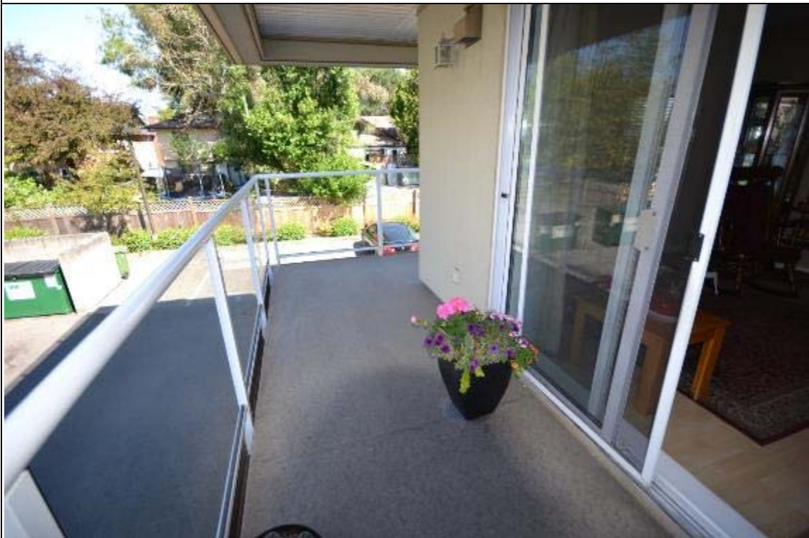
View of Typical Balcony Membrane
