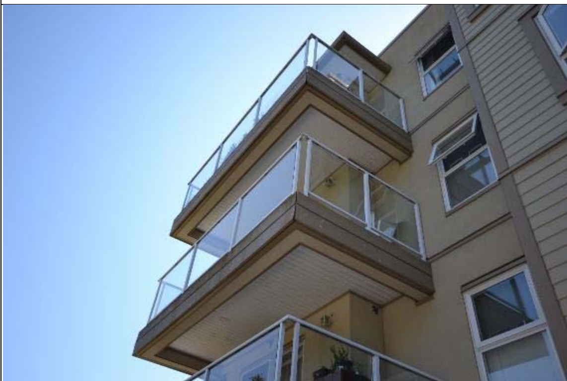
View of Balconies
