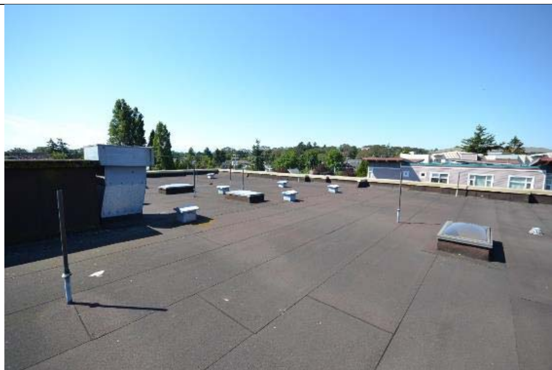
View of Roof
