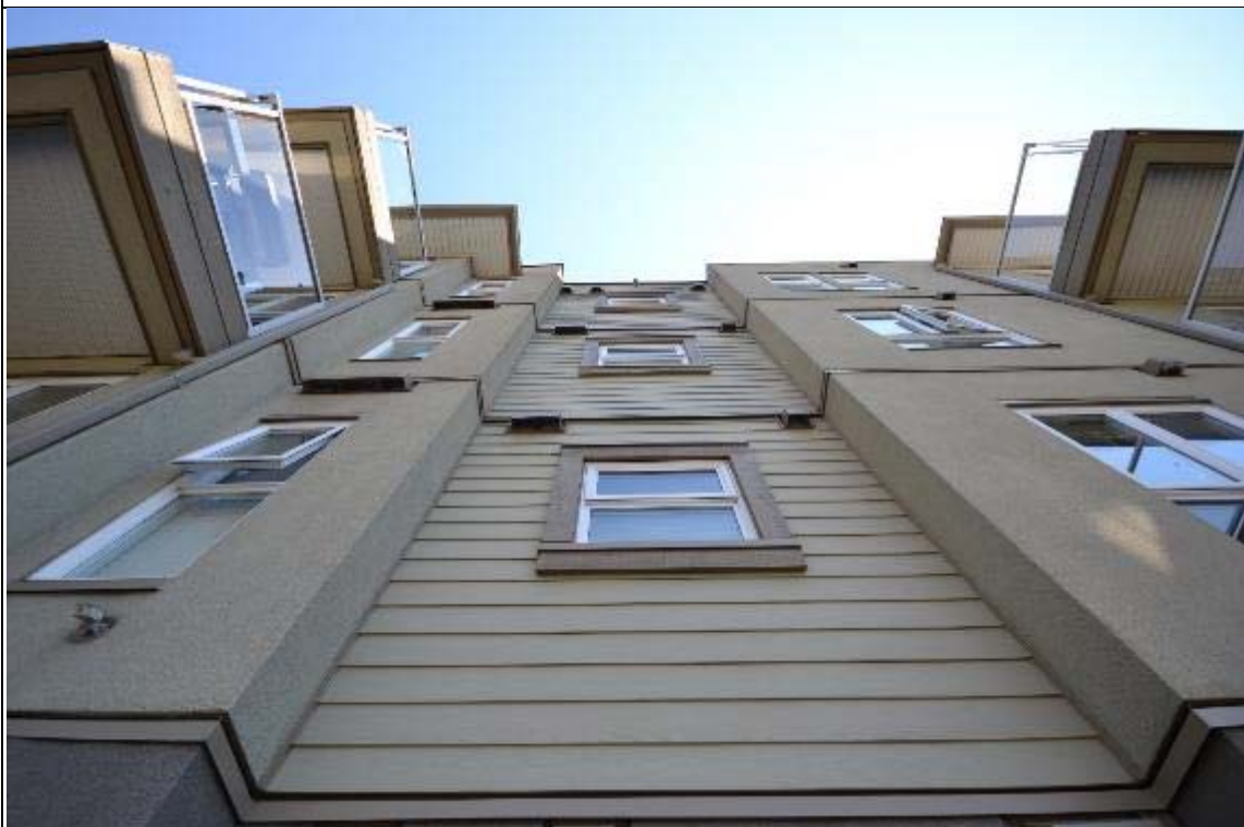
View of Fibre Cement Siding
