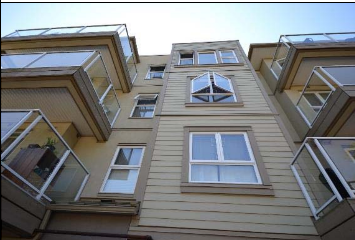
View of Typical Window Assemblies
