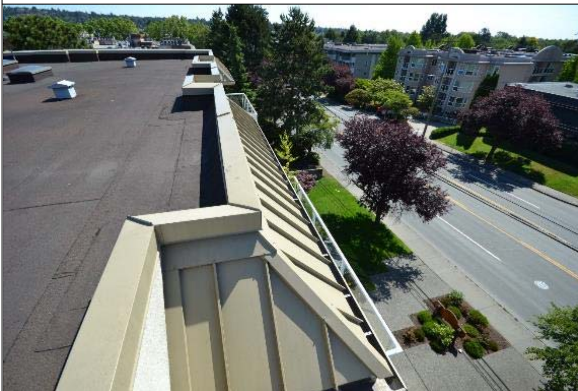
View of Roof
