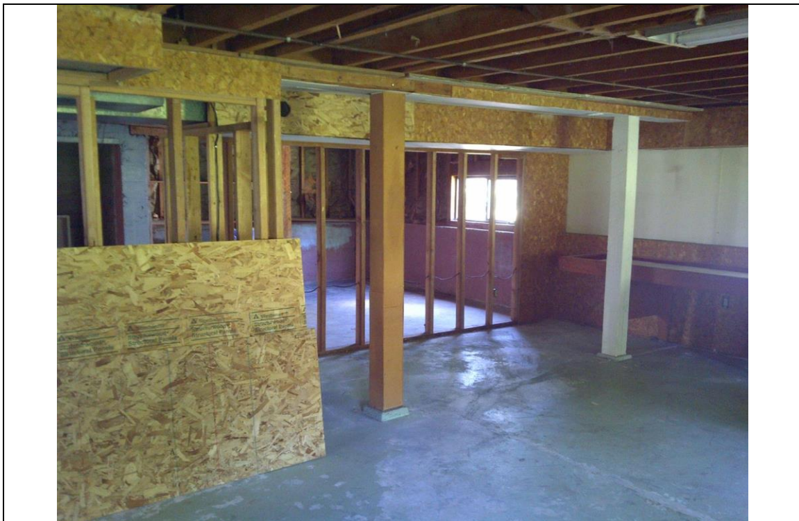
Photo 1 Date: June 7, 2013 Location: Basement Description: Green paint sampled from the floor was found to contain elevated levels of lead
