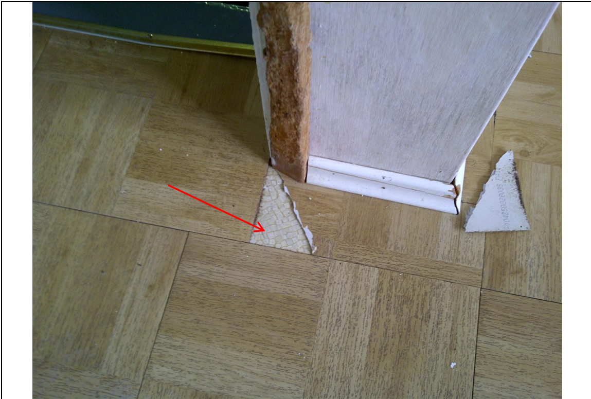
Photo 1 Date: June 7, 2013 Location: Kitchen Description: Underlying layer of vinyl sheet flooring was found to contain asbestos
