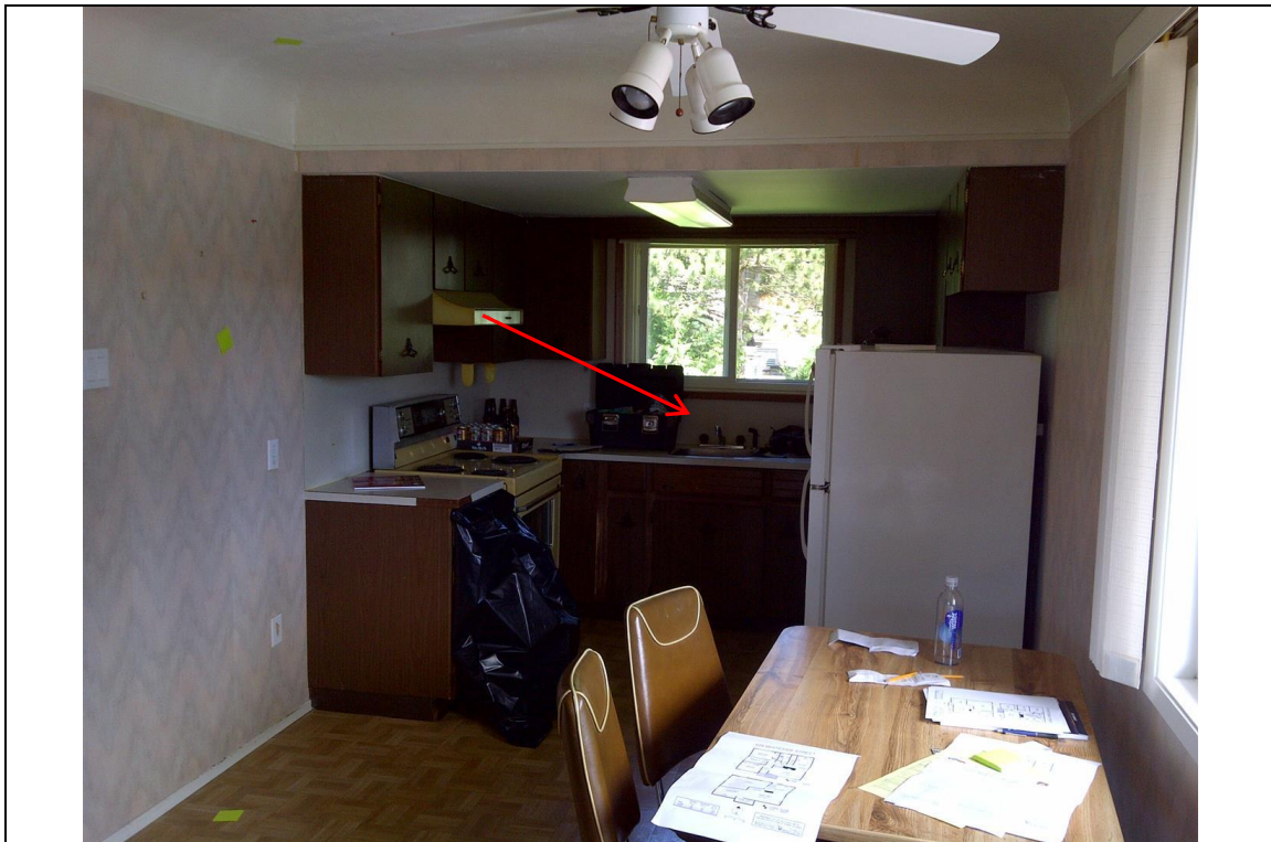
Photo 1 Date: June 7, 2013 Location: Kitchen Description: Paint sampled from the back wall was found to contain elevated levels of lead
