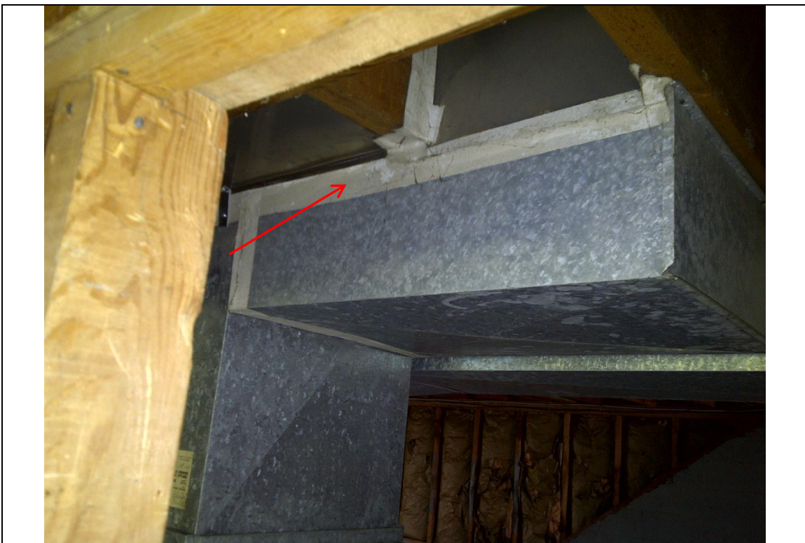
Photo 2 Date: June 7, 2013 Location: Basement Description: Furnace duct tape was found to contain asbestos
