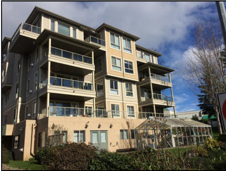
Photo No. 3: South Elevation
