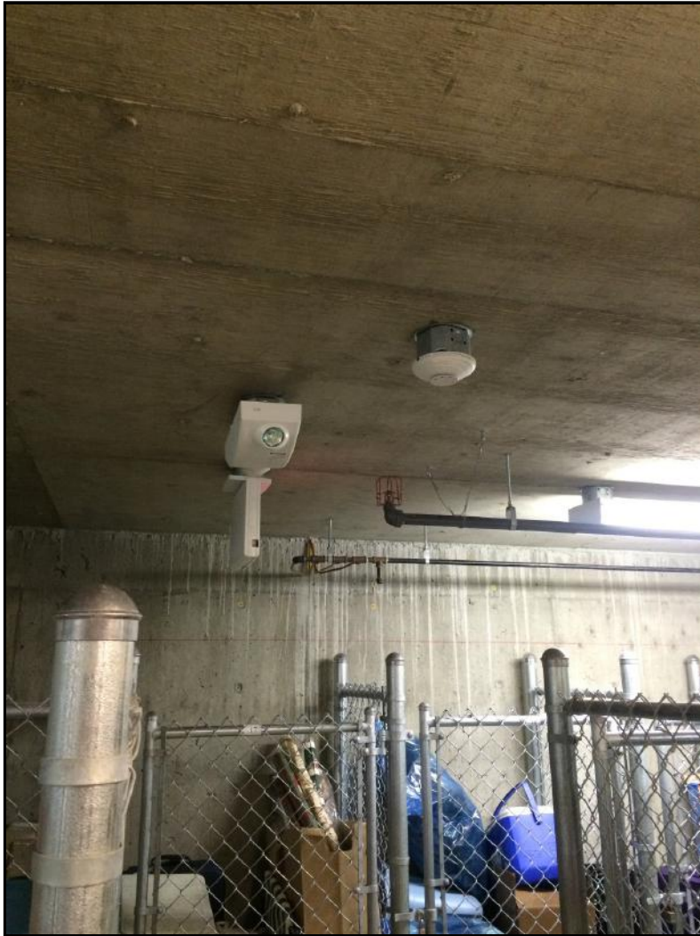
Photo No. 21: Lighting Emergency
