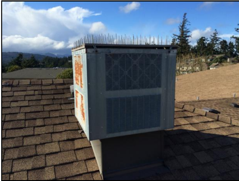
Photo No. 33: Air Handling Unit
