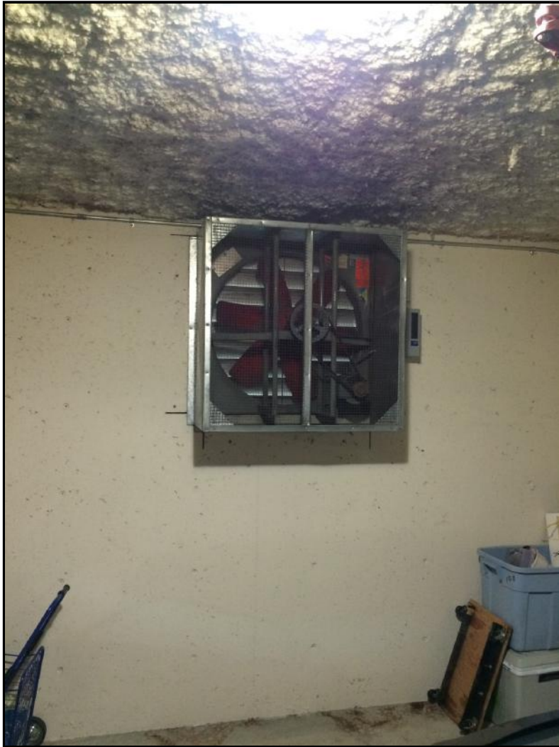
Photo No. 34: Parkade Exhaust
