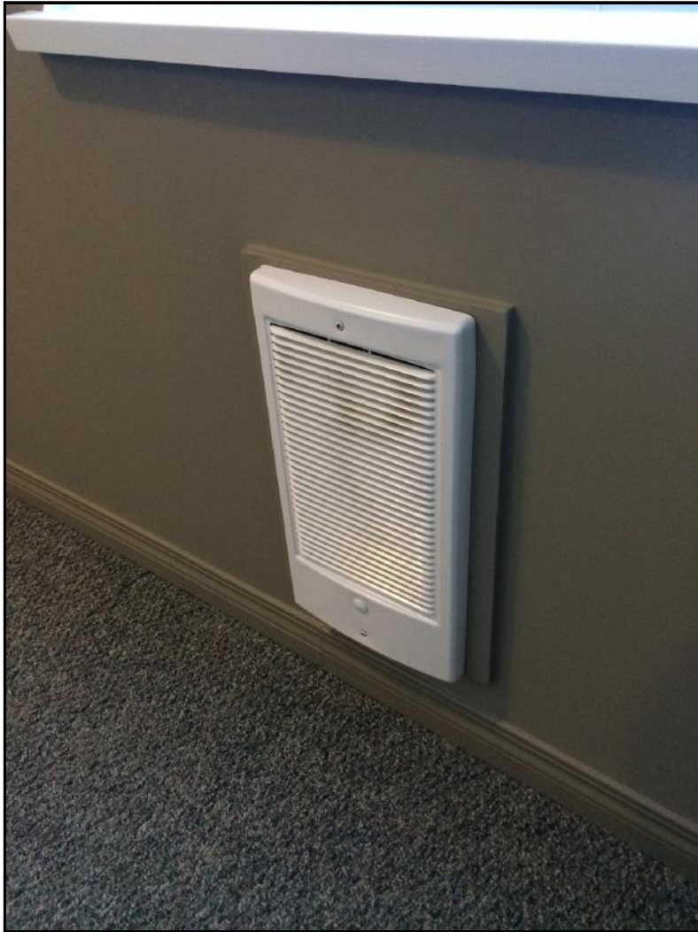
Photo No. 38: Corridor Electric Wall Heaters
