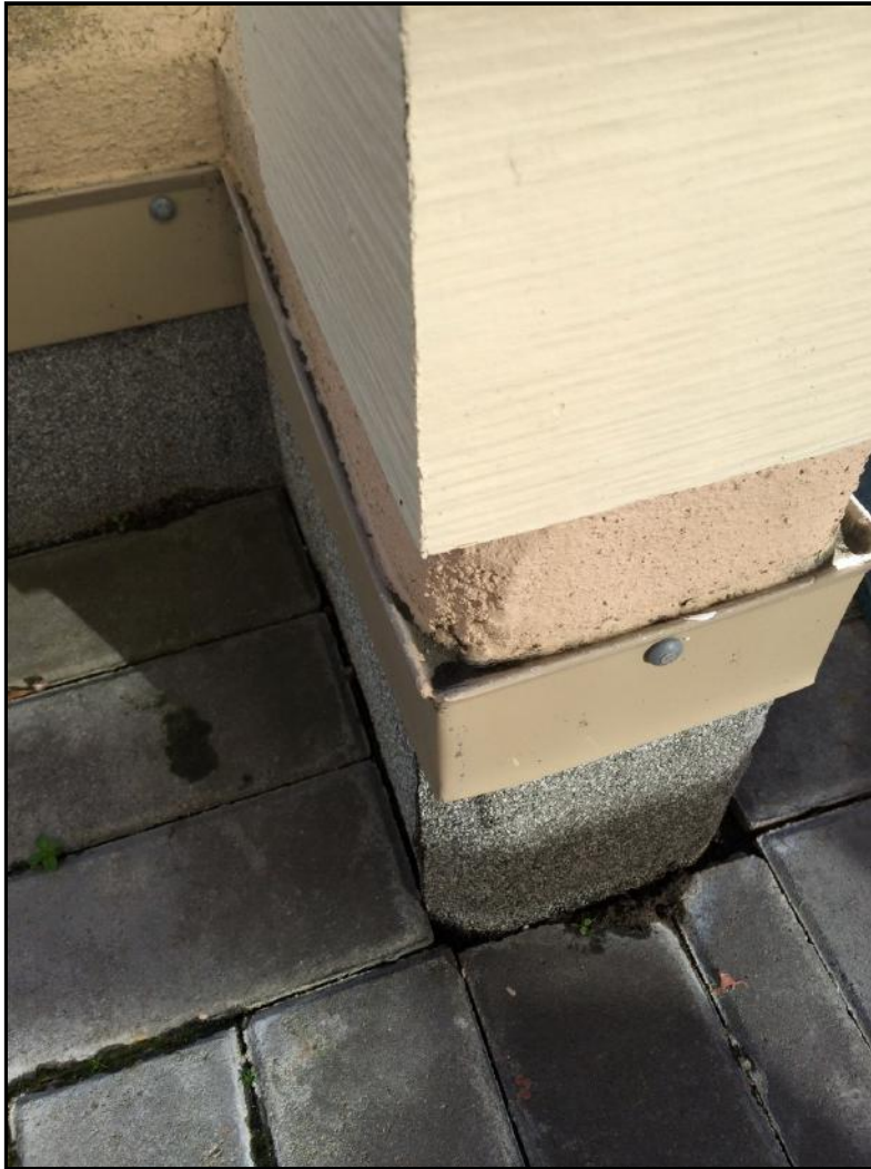
Photo No. 17: Patio Waterproofing - Over Conditioned Living Space
