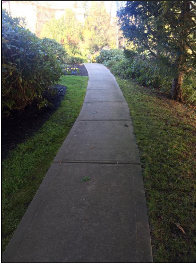
Photo No. 28: Concrete Walkways
