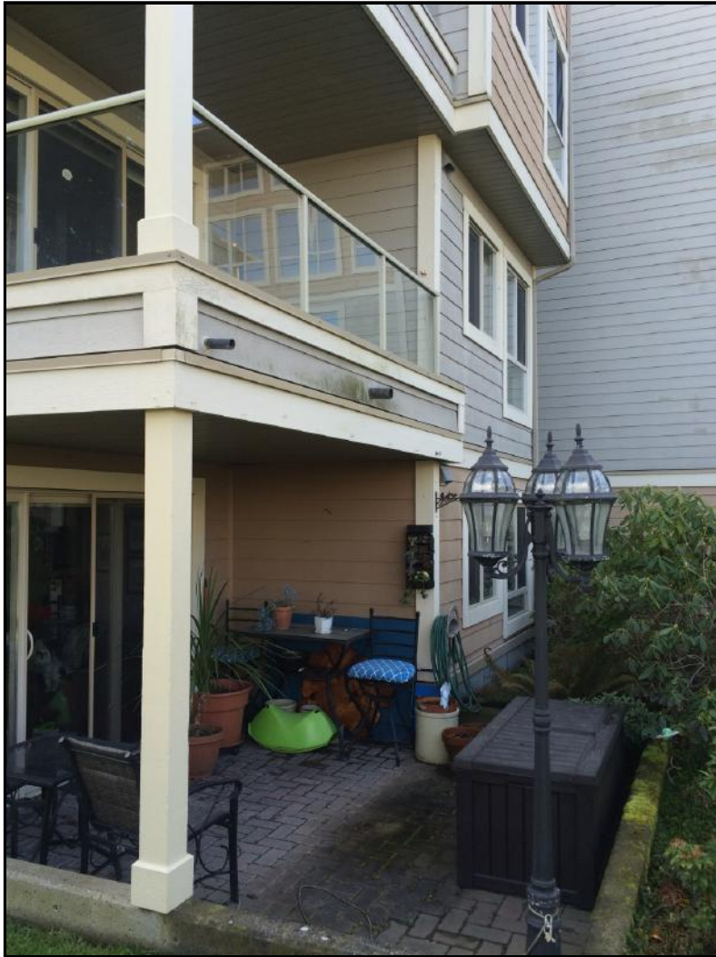
Photo No. 7: Balcony Posts
