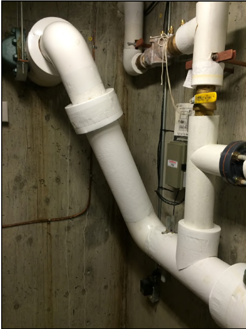
Photo No. 32: Domestic Piping
