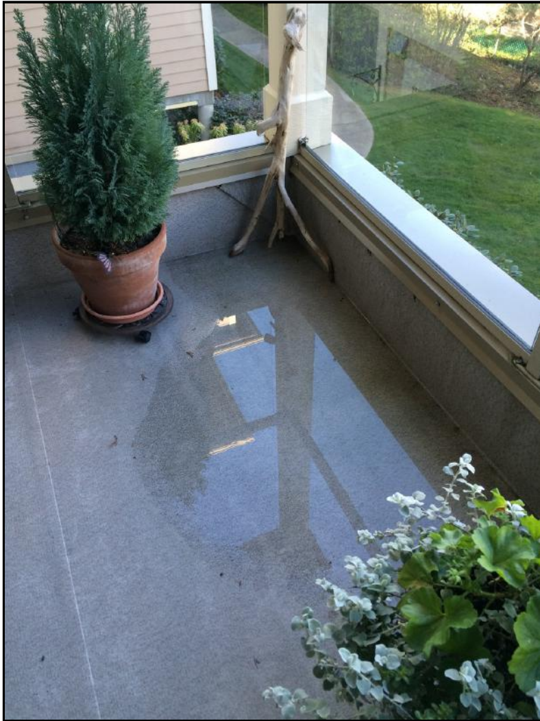
Photo No. 8: Balcony Waterproofing
