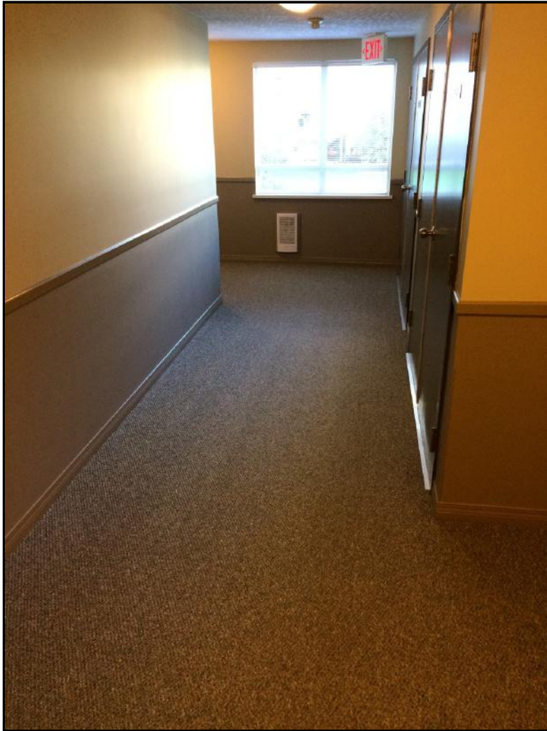
Photo No. 22: Common Area Carpeting
