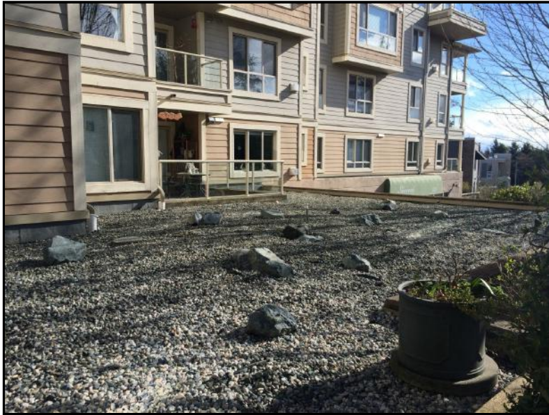
Photo No. 9: Parkade Roof Membrane
