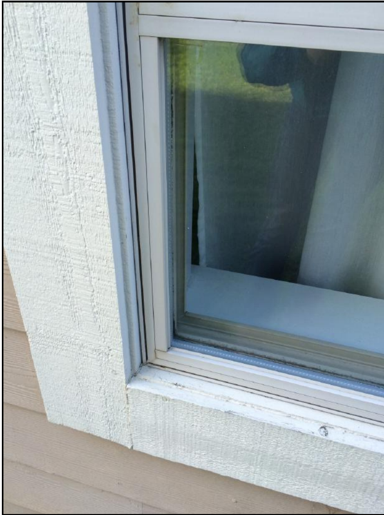
Photo No. 15: Caulking - Fenestration Sealing
