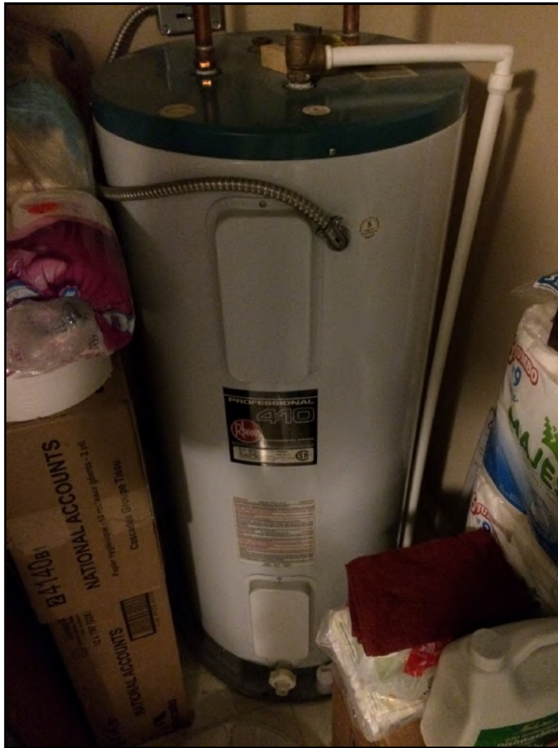
Photo No. 37: Electric Hot Water Tank
