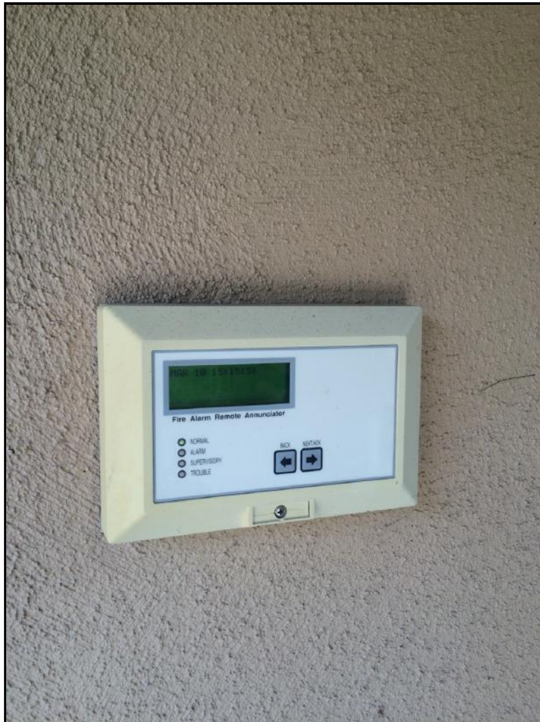
Photo No. 20: Fire Alarm System
