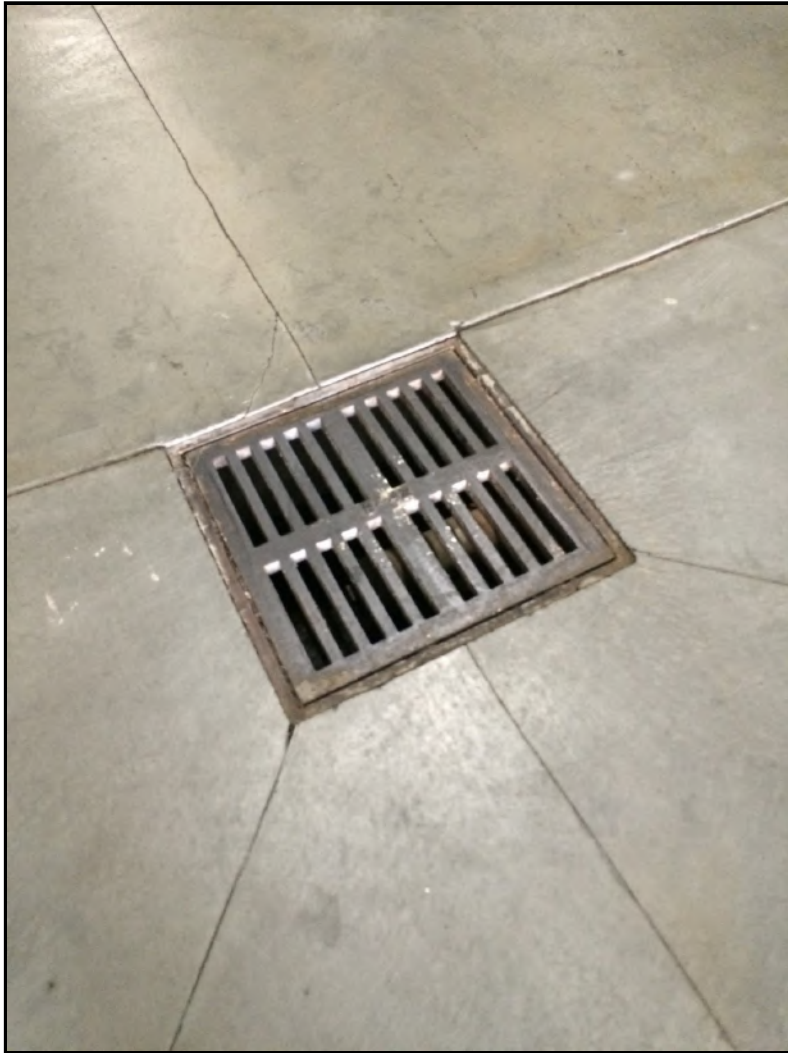
Photo No. 35: Storm Drain
