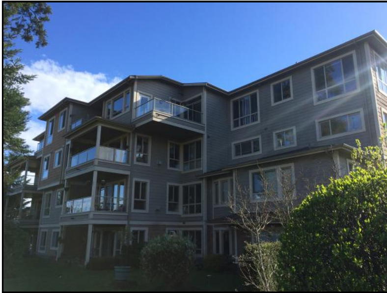
Photo No. 1: North Elevation
