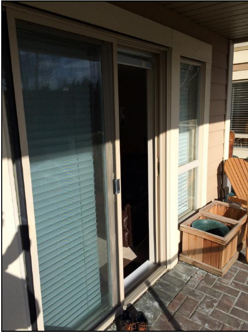
Photo No. 5: Balcony Doors
