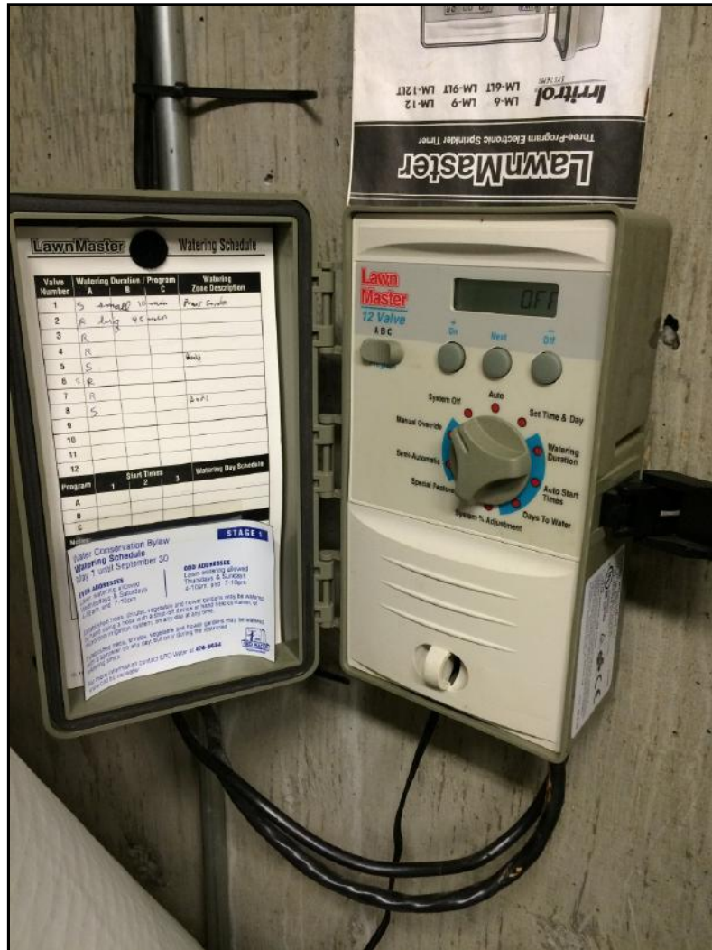
Photo No. 31: Irrigation Controls
