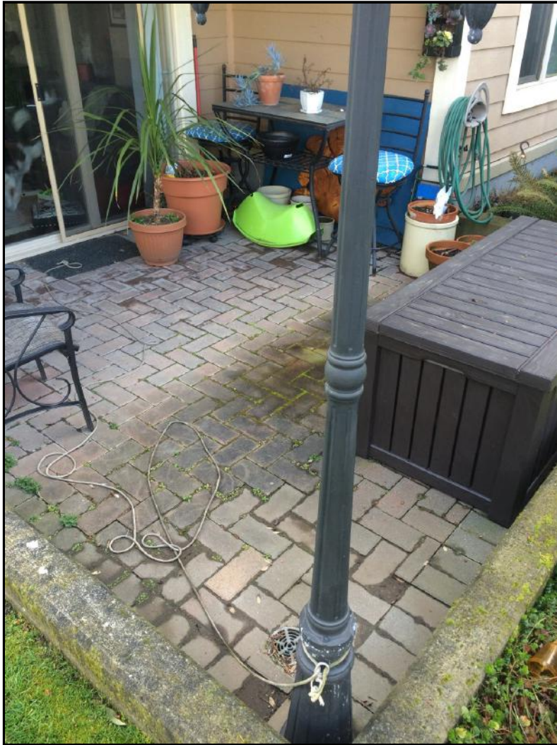
Photo No. 29: Patio Pavers
