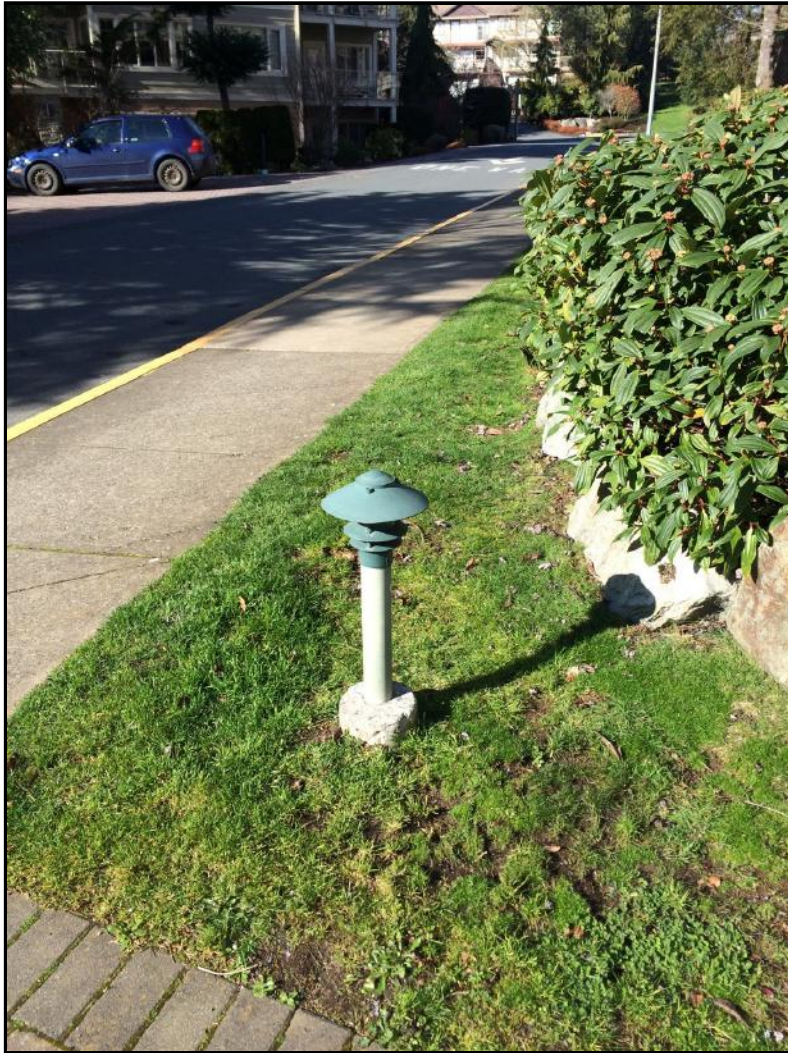
Photo No. 36: Exterior Lighting
