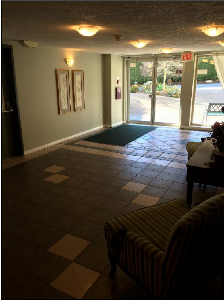
Photo No. 23: Lobby and Parkade Vestibule Flooring
