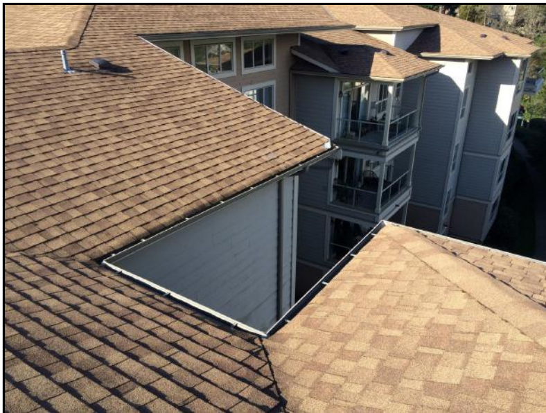
Photo No. 19: Metal Gutters
