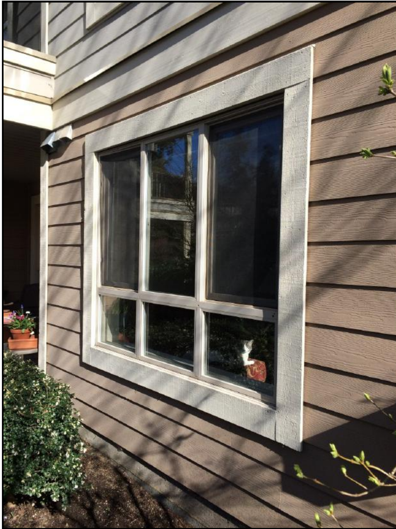
Photo No. 14: Vinyl Windows - H Coupler
