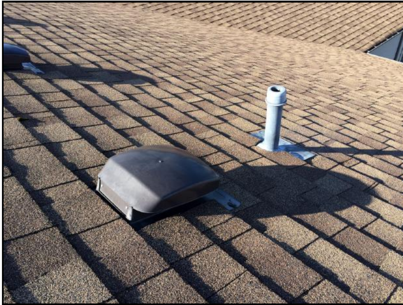
Photo No. 18: Asphalt Shingles
