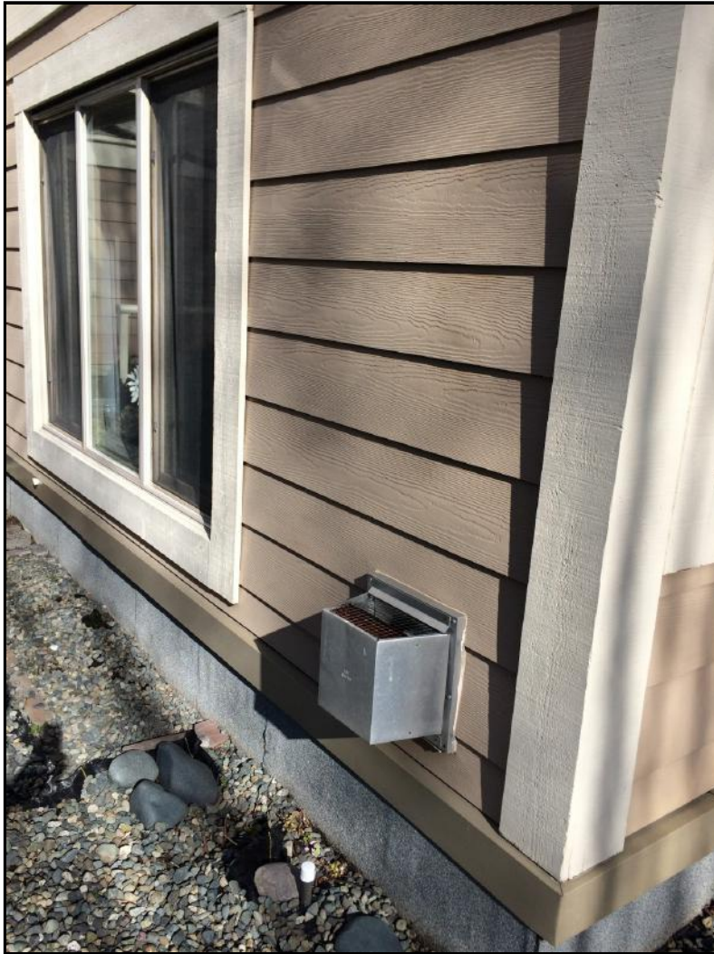
Photo No. 12: Fiber Reinforced Concrete (FRC) Siding
