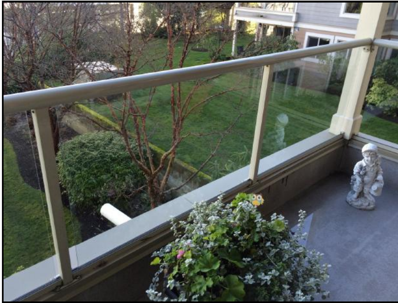
Photo No. 6: Balcony Railings
