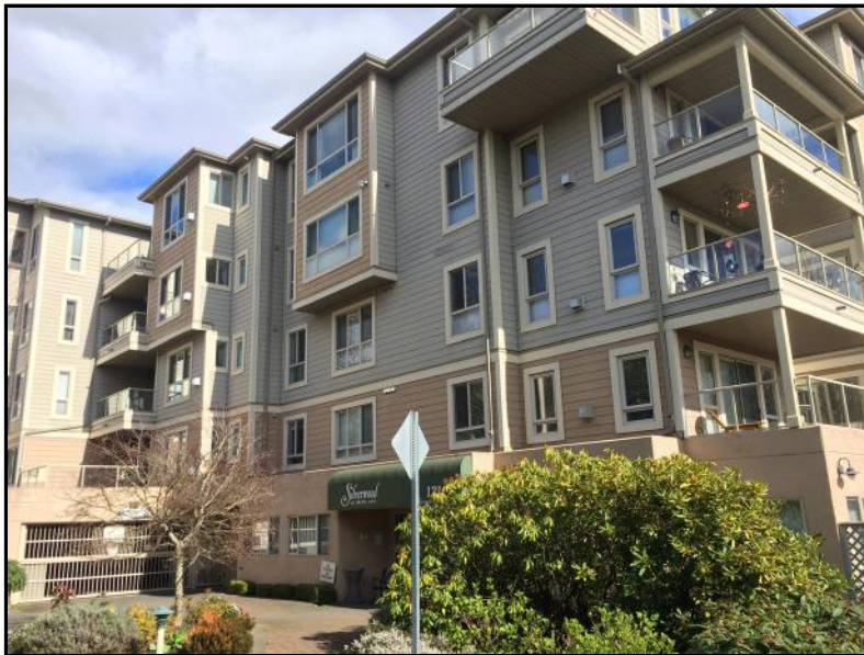
Photo No. 4: West Elevation
