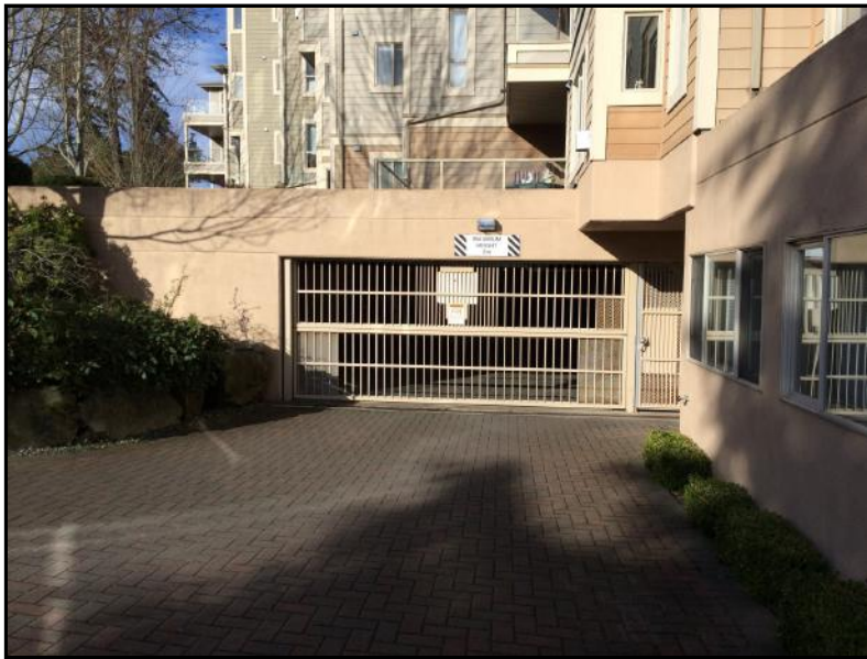
Photo No. 10: Parkade Gate
