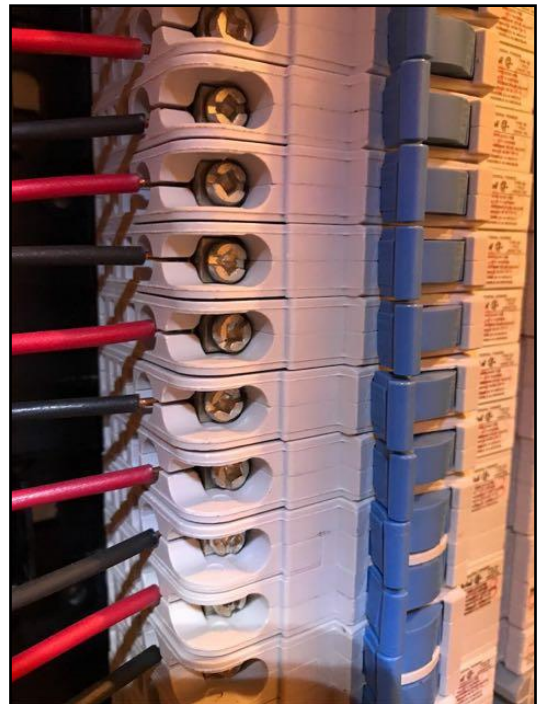
79. Copper - non-metallic sheathed
