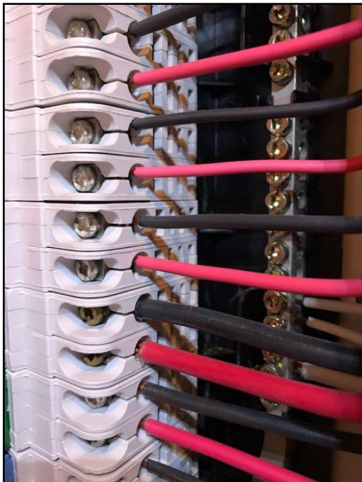
78. Copper - non-metallic sheathed
