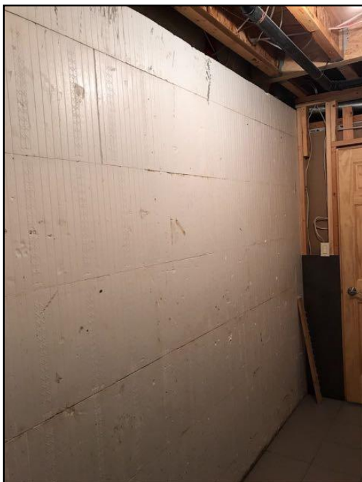
61. Insulating concrete forms
