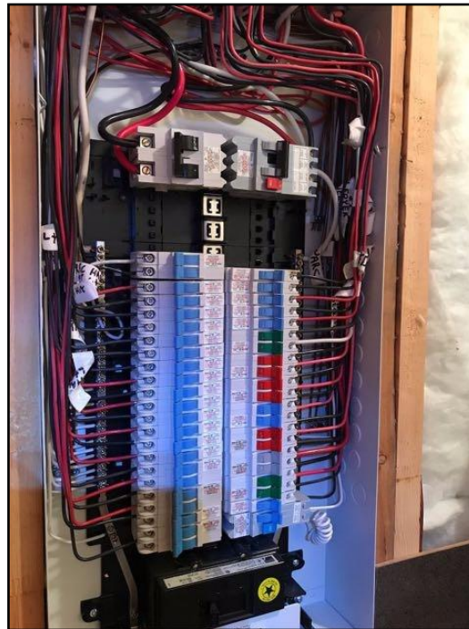
69. Breakers - utility room
