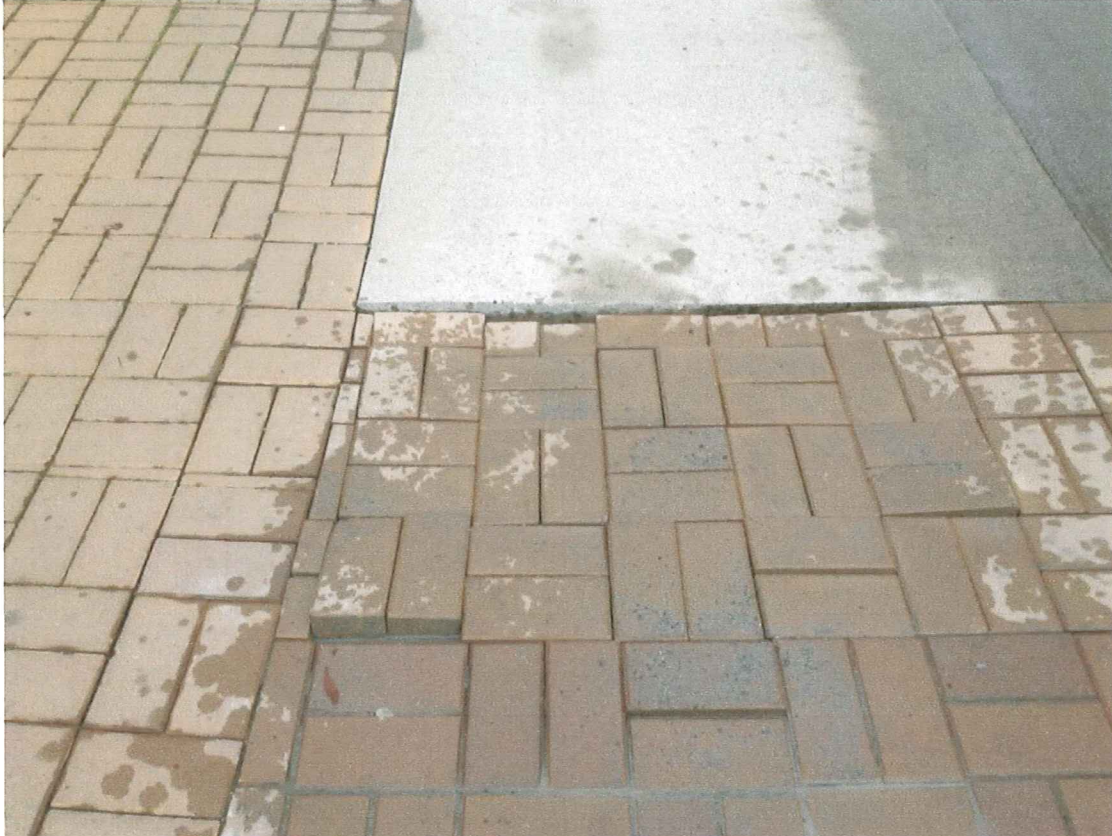
Figure 3, Close up view of brickwork with groundwater extrusion.
