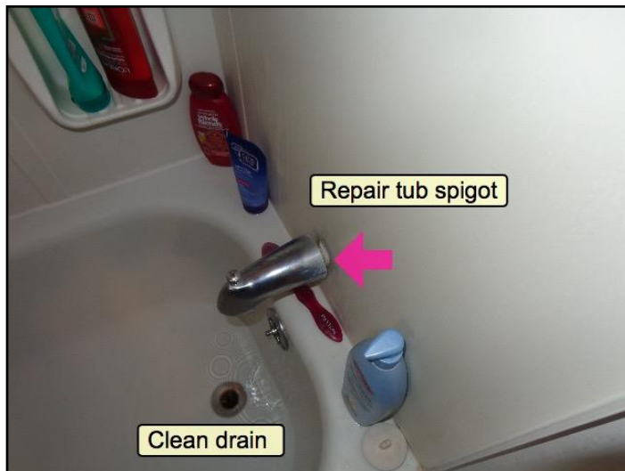
18. Clean drain, repair tub spigot
