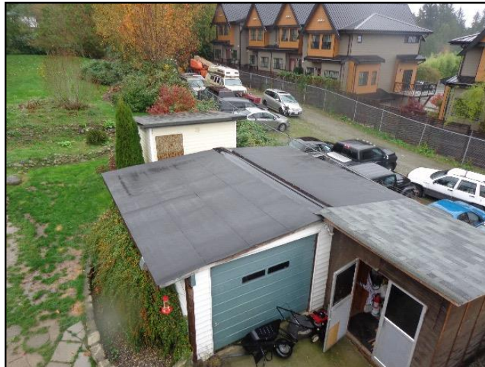
1. Modified bitumen membrane
