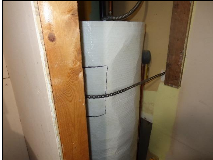
21. Water heater in blanket
