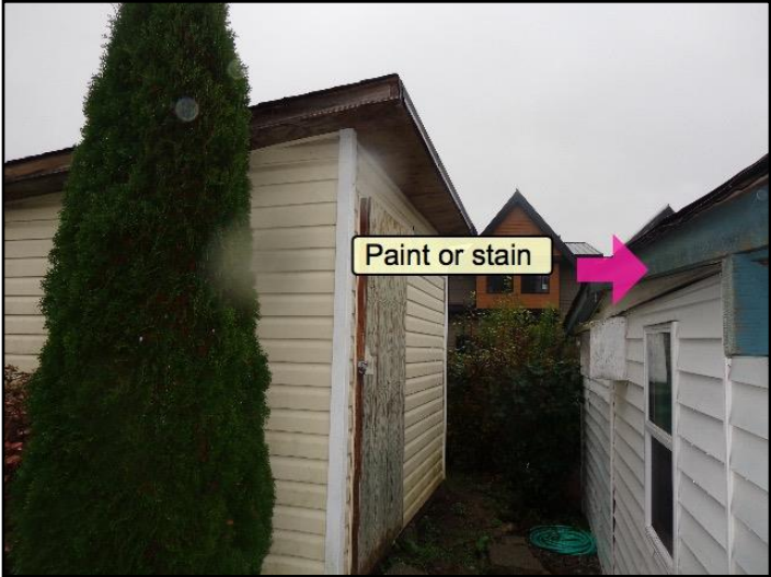
7. Paint or stain needed
