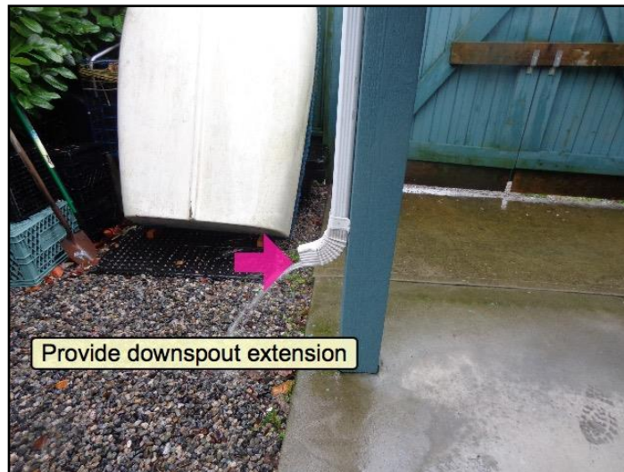
6. Should discharge 6 feet from building
