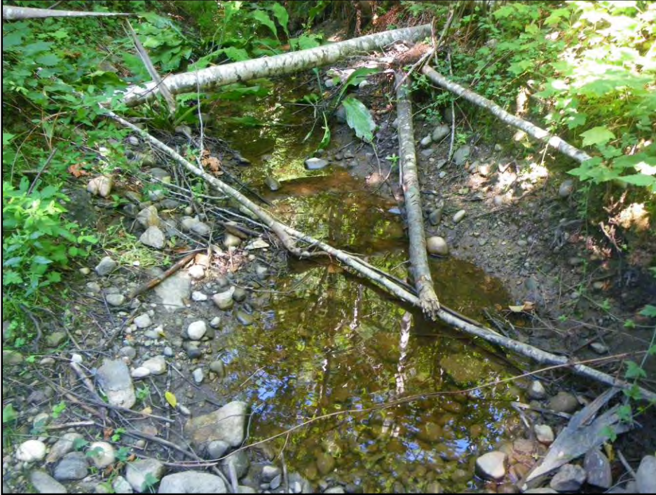
Residual standing water located at the current gravel road crossing on Jordans Creek (Reach 1). Pacific tree- frog tadpoles were observed in this pool during the field assessment.
