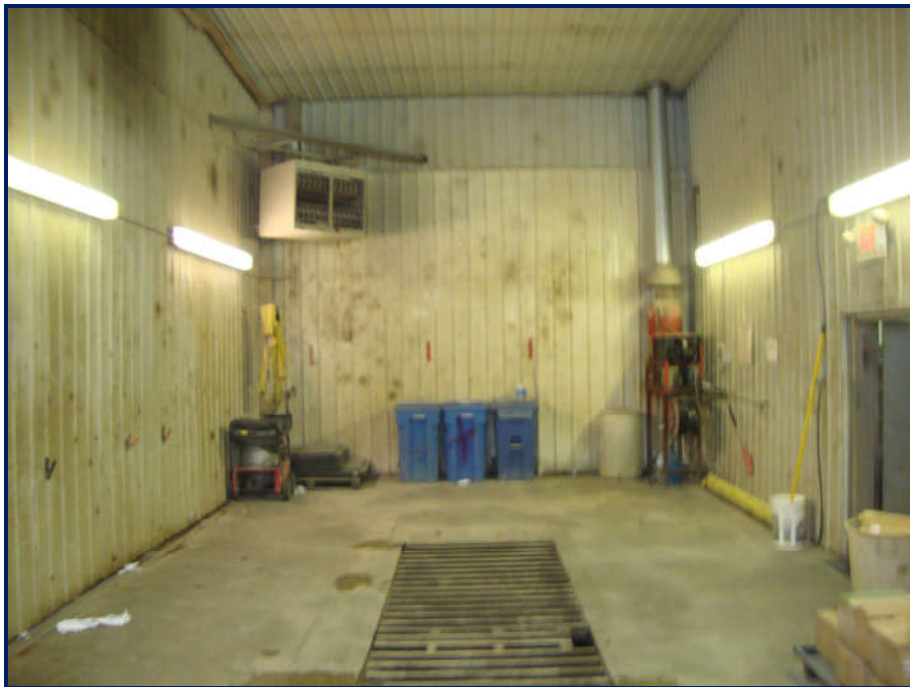
Wash Bay – Looking South
