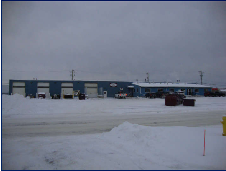
Front View of Subject Property – Looking South
