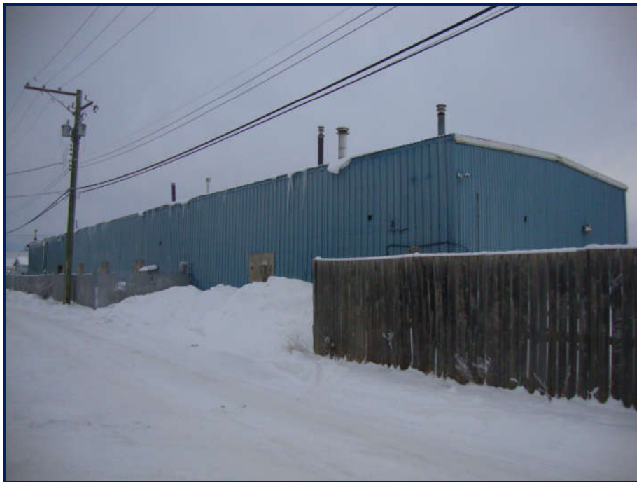
Rear View of Subject Property – Looking Northwest
