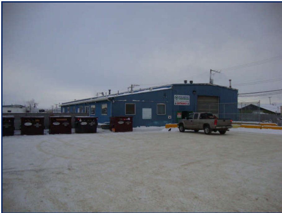
Front View of Subject Property – Looking Southeast
