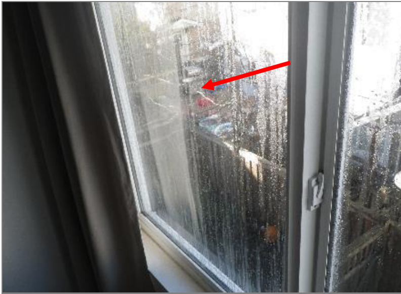
Figure 2.11 Condensation on the interior surface of glass. Photo taken at the bay at the master bedroom of suite 70.
