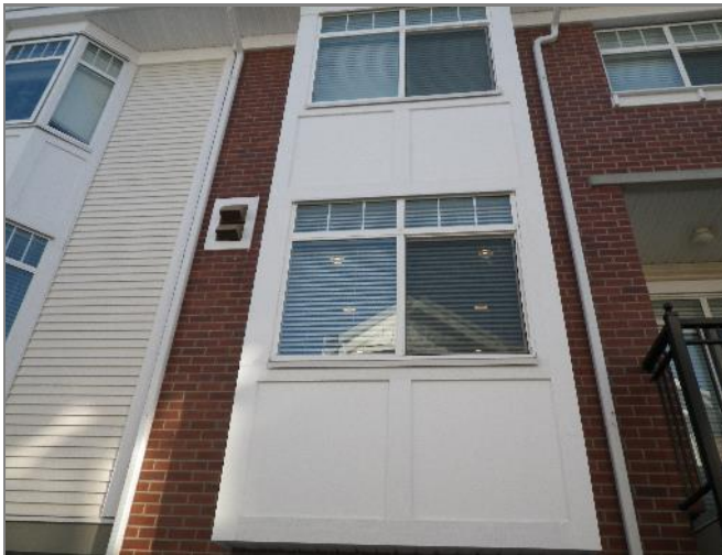
Figure 2.1 Photo of a typical bay at Manhattan Skye.
