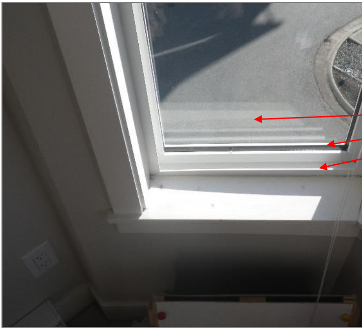
Figure 2.8 Photo of bay assembly taken at interior of suite 83, south elevation. IGU Swiggle spacer (black) Sill track
