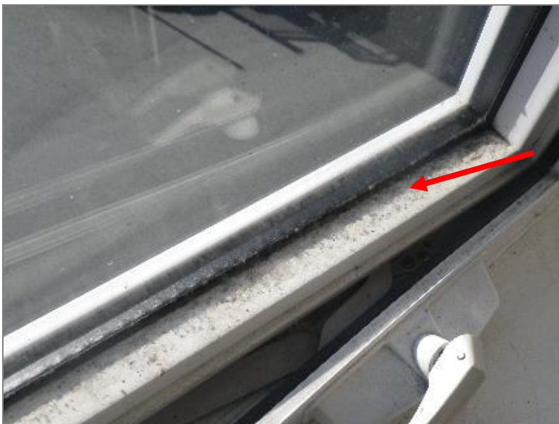
Figure 2.13 Staining & mould on the window frame of casement vent of bay window. Photo taken at master bedroom window of suite 31.
