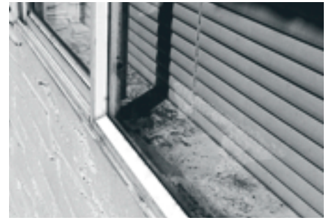
Evidence of problems resulting from condensation can be seen on the interior window sill.
