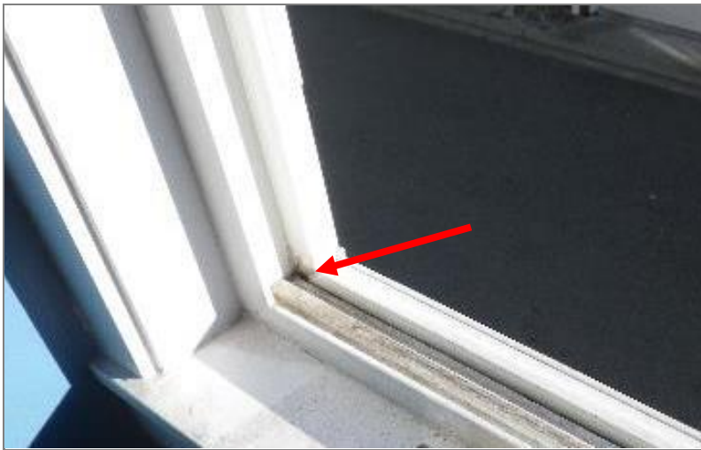
Figure 2.12 Staining & mould on the window frame within slider vent track at a bay. Photo taken at kitchen window at suite 70.
