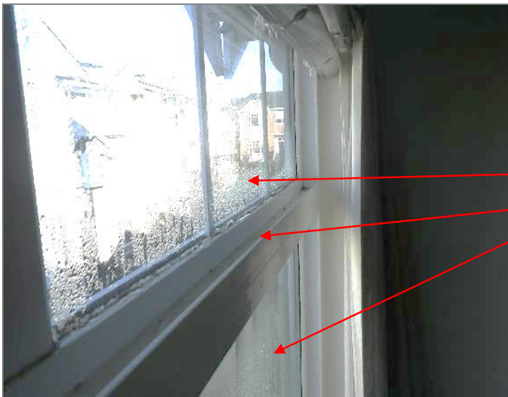
Figure 2.10 Photo of bay assembly taken at interior of suite 70. IGU Secondary track IGU
