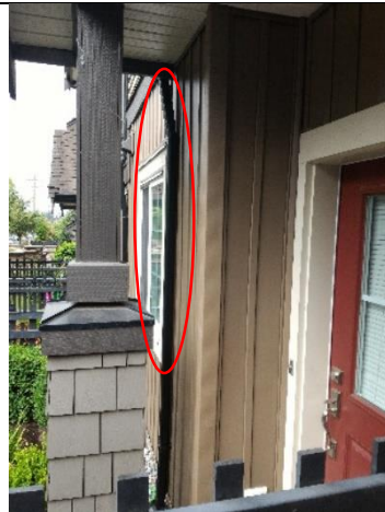
Siding corner trim show uneven surface. This is an aesthetic concern only, the performance of the siding will not be affected.
