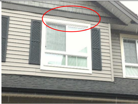
Siding has dislodged at unit 57.
