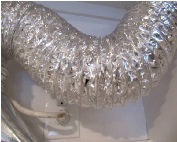
Fix the hole in the range vent.
