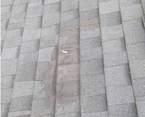
Patch work noted on the main roof above the water staining in the attic.
