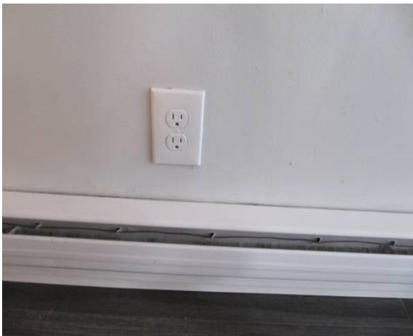
Outlets over baseboards aren't recommended.
