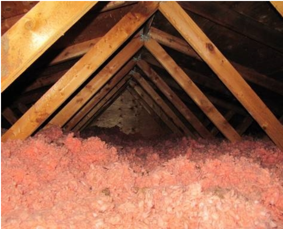
General view of the attic.
