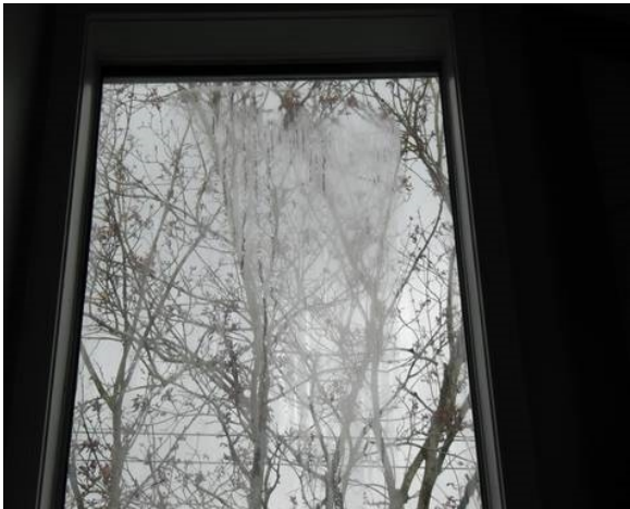
Failed seal between windows.
