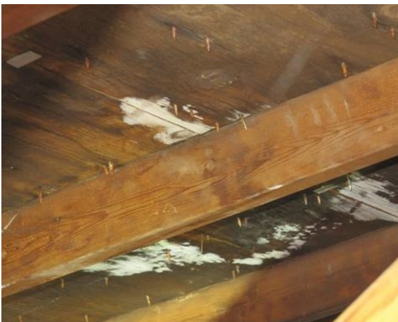
Water stains noted in the attic.
