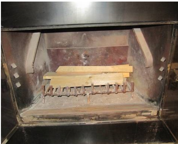
General view of the wood burning fireplace.
