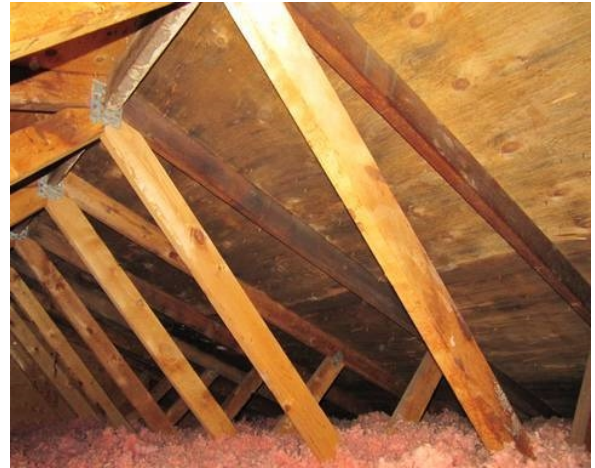
Minor staining noted in the attic.
