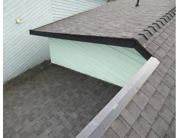
General view of the roof.
