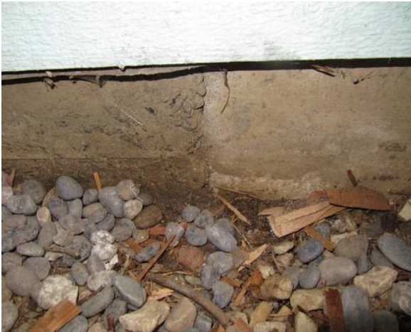
Minor foundation crack.
