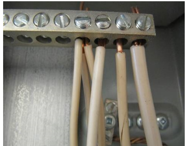
Neutral wires should have their own spot, not 3 in one spot.
