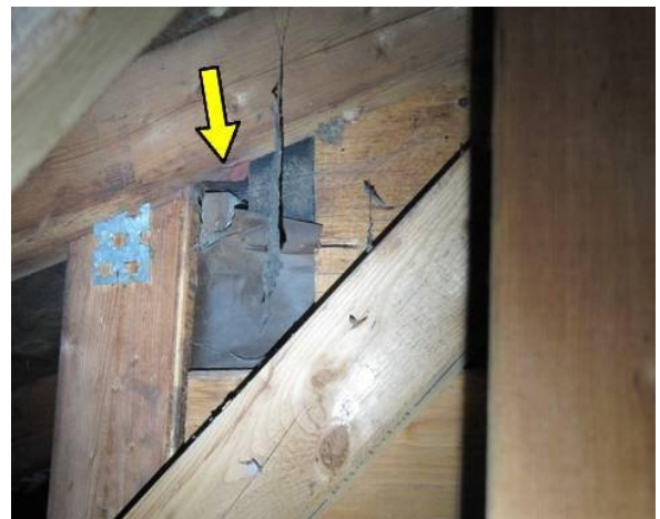
Holes in the attic need to be sealed.
