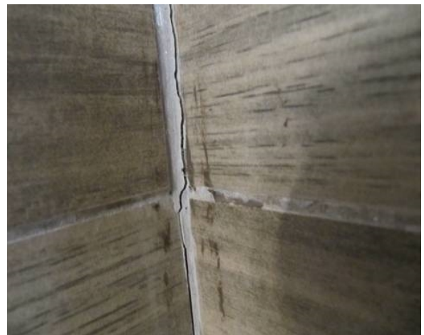
Grout cracks should be repaired.
