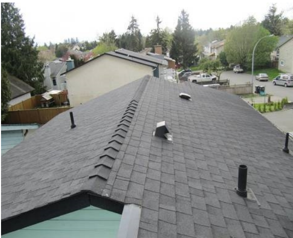
General view of the roof.
