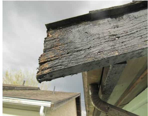
Fascias are deteriorating.
