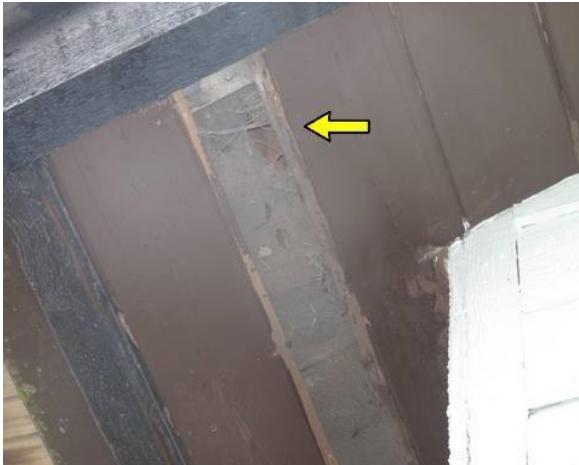
Fix holes in soffit vents.
