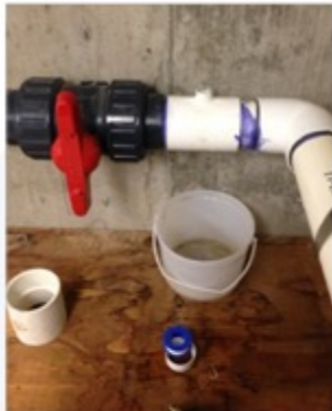
New well pump house piping
