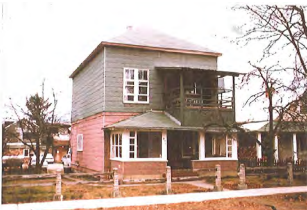
Residential Rehabilitation project transforms low income rental unit to offices for forest technology consulting firm.
