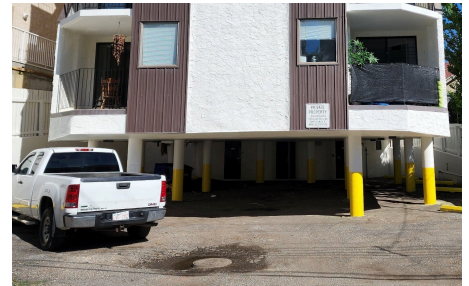
Rear elevation — balconies and covered parking.
