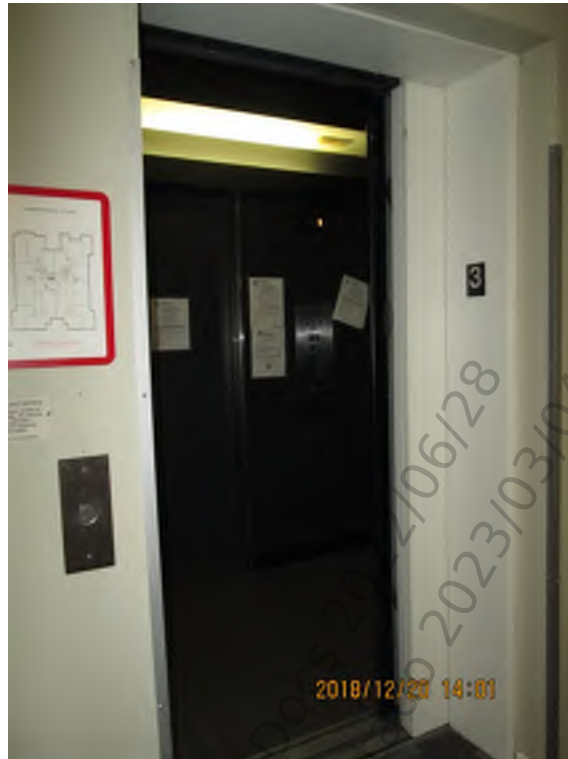
Photo 5 – Floor 3 lobby view
