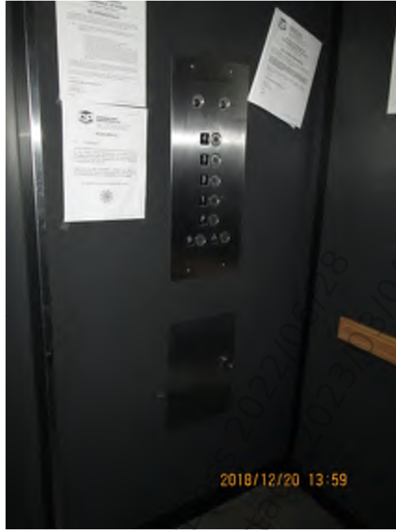
Photo 3 - Elevator car station
