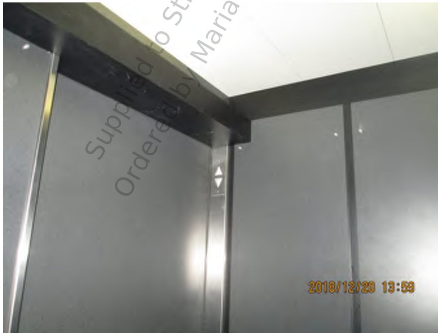
Photo 4 - Elevator cab finishes
