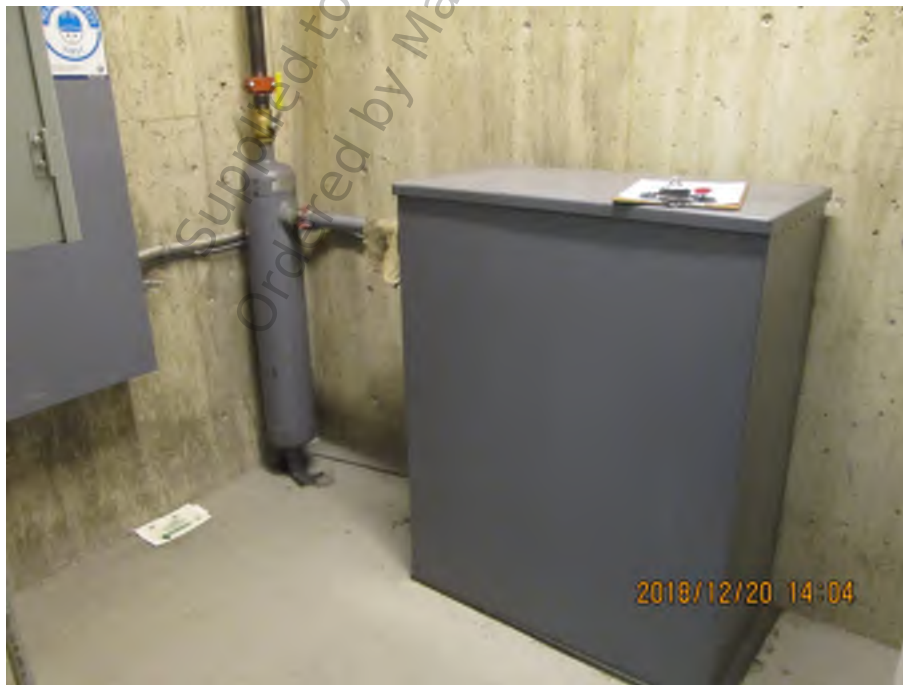
Photo 2 - Elevator hydraulic pumping unit
