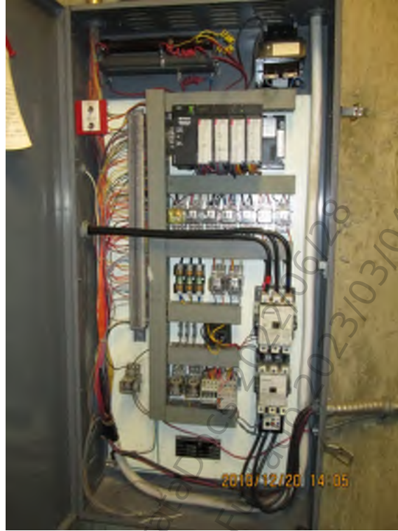
Photo 1 - Elevator controller
