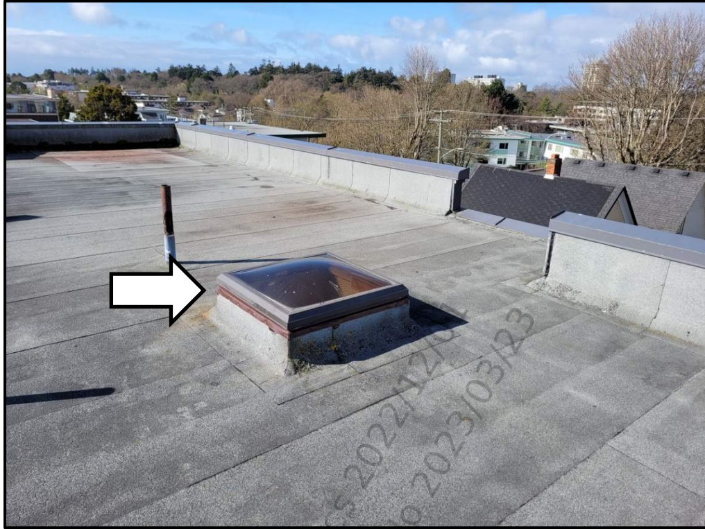
Photo 7 (B20 20 99) - Skylight Roof Hatch Cover
