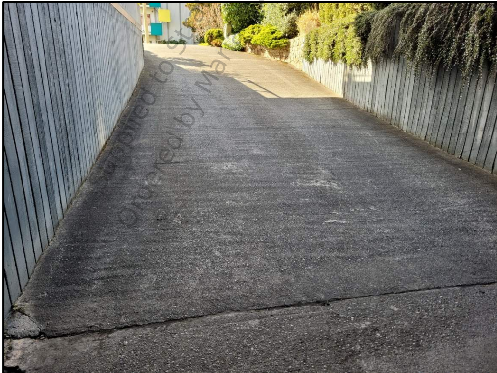
Photo 36 (G20 10 00) - Concrete Pavement at Parkade Ramp
