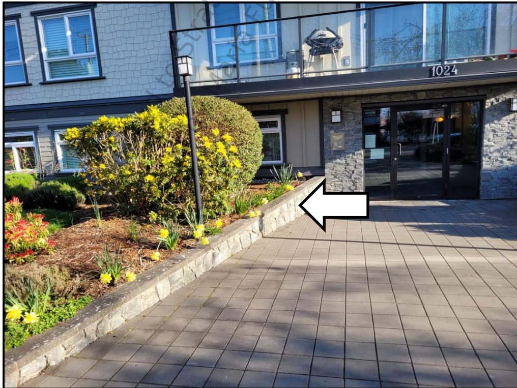
Photo 40 (G20 40 01.03) - Stone Masonry Retaining Walls Leading to Front Entrance
