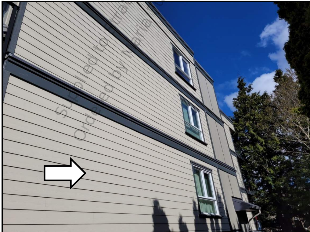
Photo 4 (B20 10 00.01) - Fibre Cement Cladding
