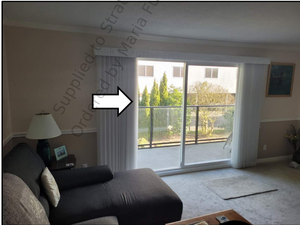
Photo 8 (B20 30 02.01) - Sliding Door at Balcony
