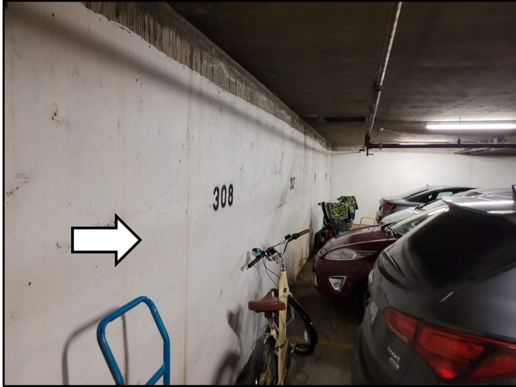
Photo 1 (A10 00 00) - Foundation Wall Viewed From Within Parkade
