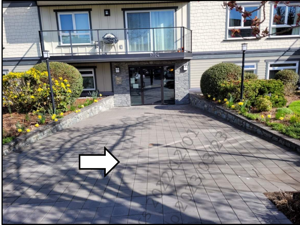
Photo 37 (G20 30 00) - Concrete Unit Pavers at Front Entrance Walkway
