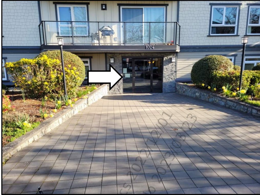
Photo 9 (B20 30 02.03) - Front Entrance Doors
