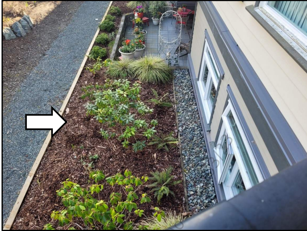
Photo 13 (B30 10 02.02) - Overburden above Podium Deck Waterproofing
