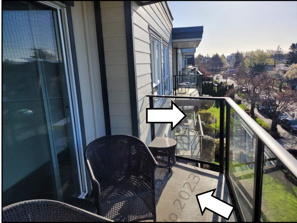
Photo 3 (B10 10 04) - Balconies, Showing Vinyl Waterproofing Membrane and Railings
