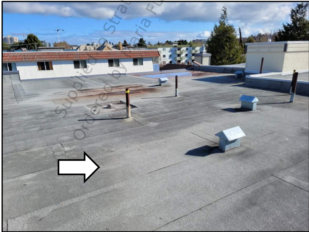
Photo 12 (B30 10 02.01) - SBS-Modified Bitumen Membrane at Main Roof
