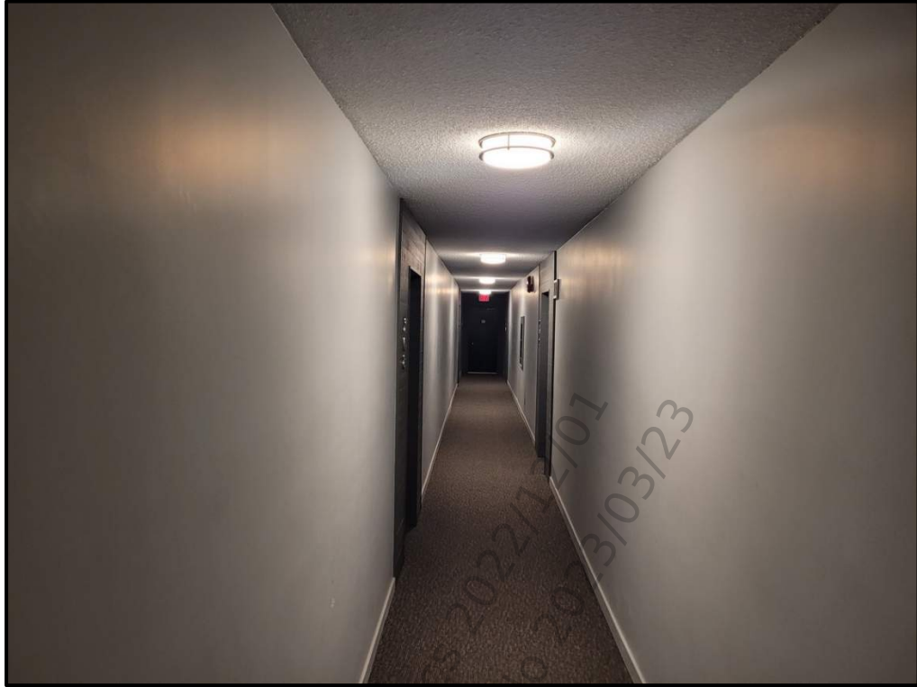
Photo 15 (C30 00 00.01) - Interior Finishes in Hallway
