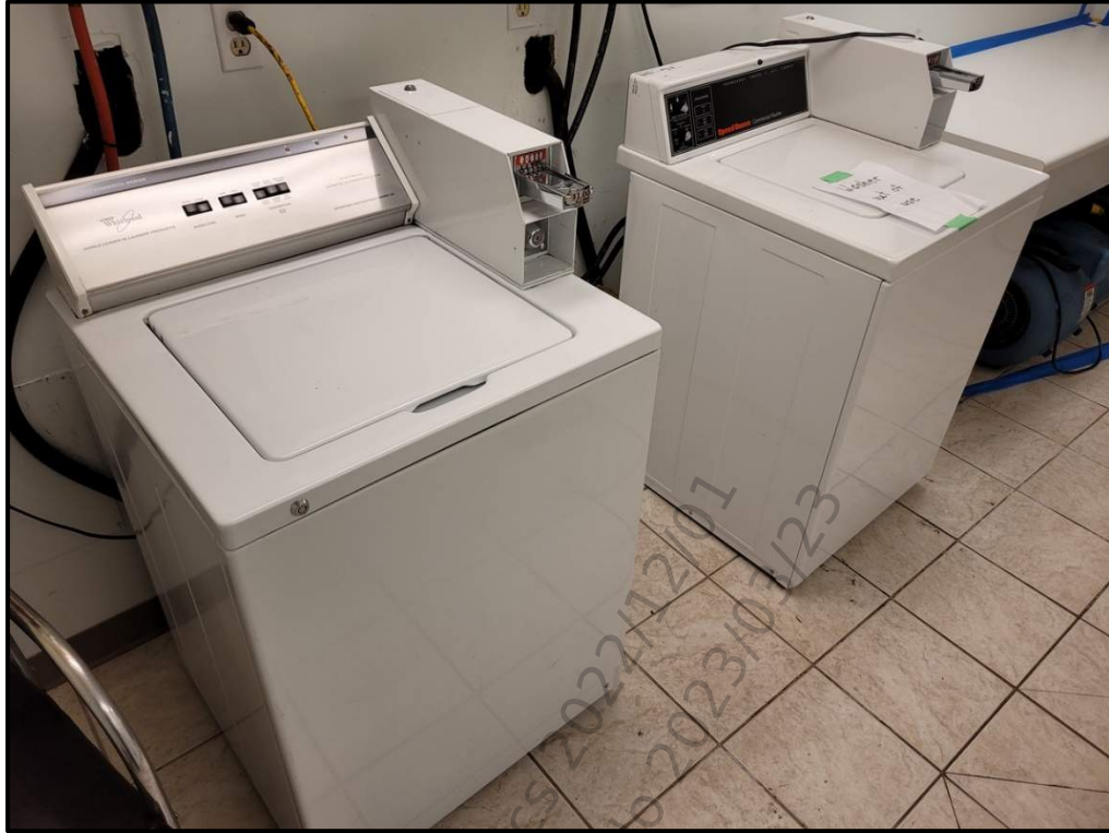
Photo 35 (E10 10 04) - Laundry Equipment
