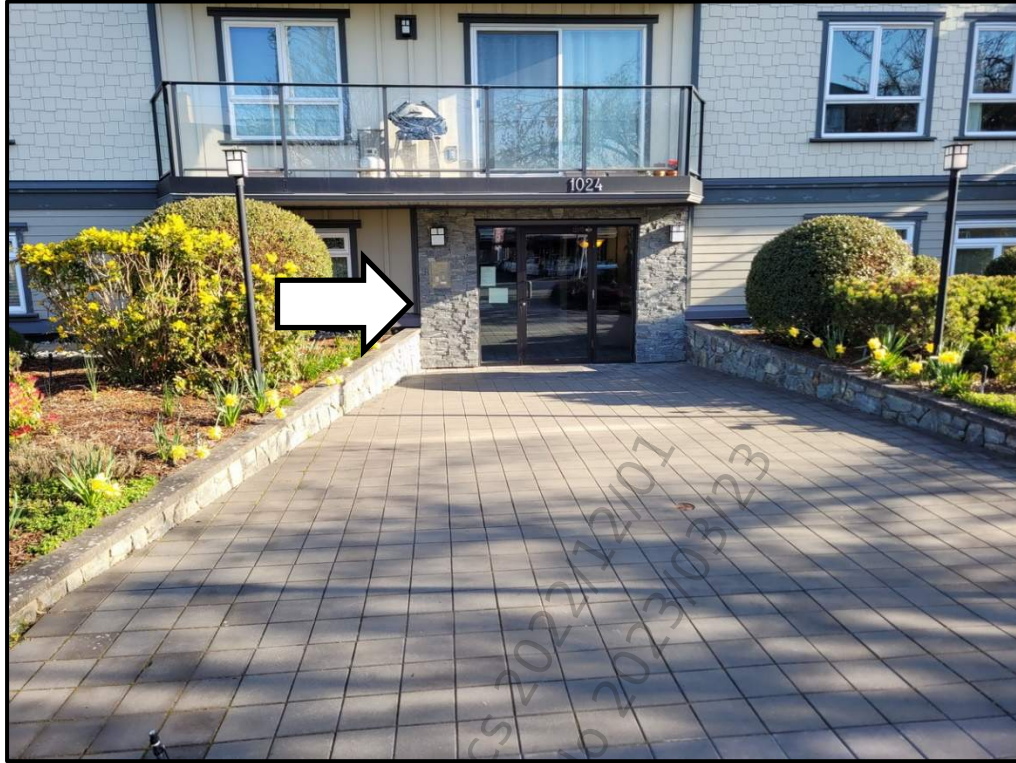
Photo 5 (B20 10 00.03) - Stone Veneer Cladding around Front Entrance
