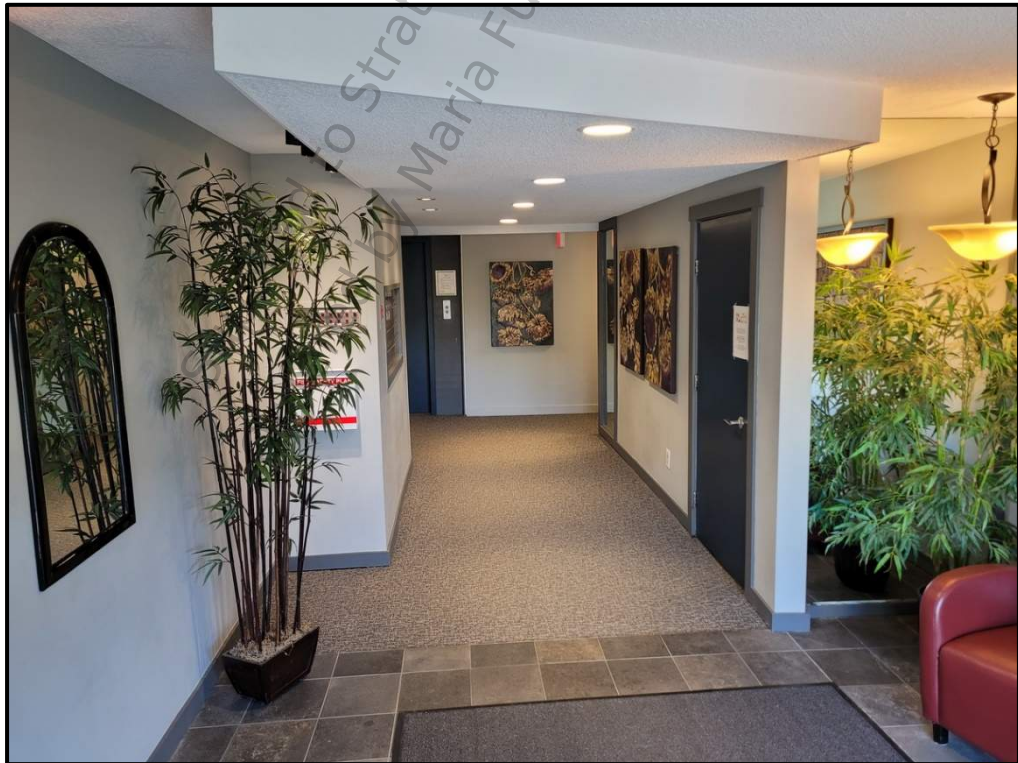
Photo 16 (C30 00 00.02) - Interior Finishes in Front Lobby
